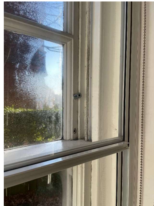
Photo 08: Consistent condensation with sign of mould
