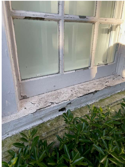
Photo 06: Deteriorating timber sill with early sign of rot
