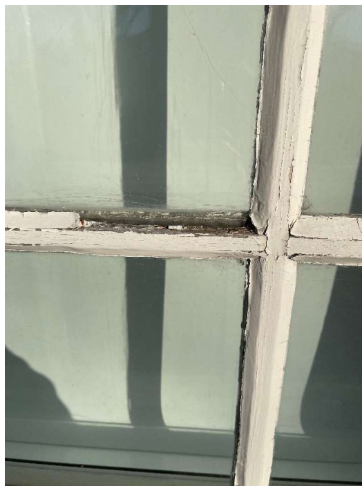
Photo 02: External peeling paint works to rear garden door
