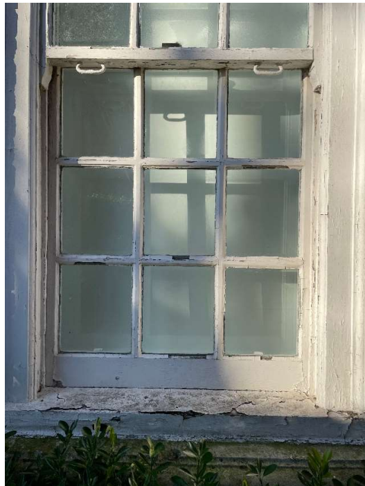
Photo 04: External frame and glazing bar condition
