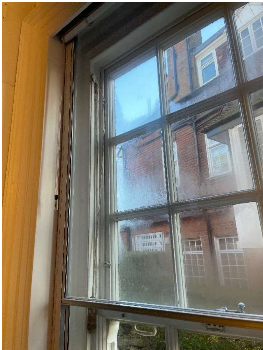
Photo 07: Internal view with secondary glazing with condensation on the inner side of primary glazing
