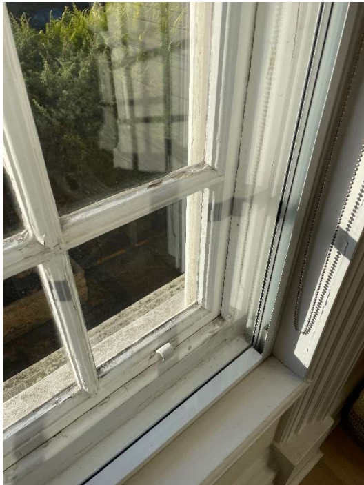
Photo 05: Existing second layer of internal glazing
