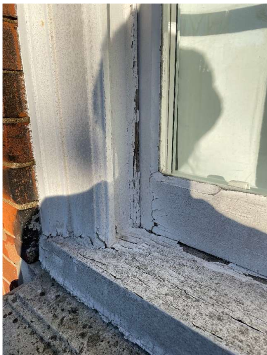
Photo 01: External peeling paint works to rear garden door
