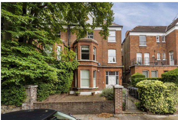
Figure 3 – Typical dwelling in Cranfield Gardens, South Hampstead Conservation Area
