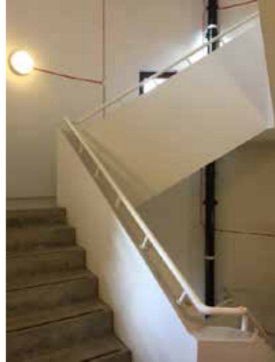
Interior of circular fire escape stair north of west wing
