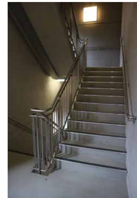
BLCC Fire escape staircase
