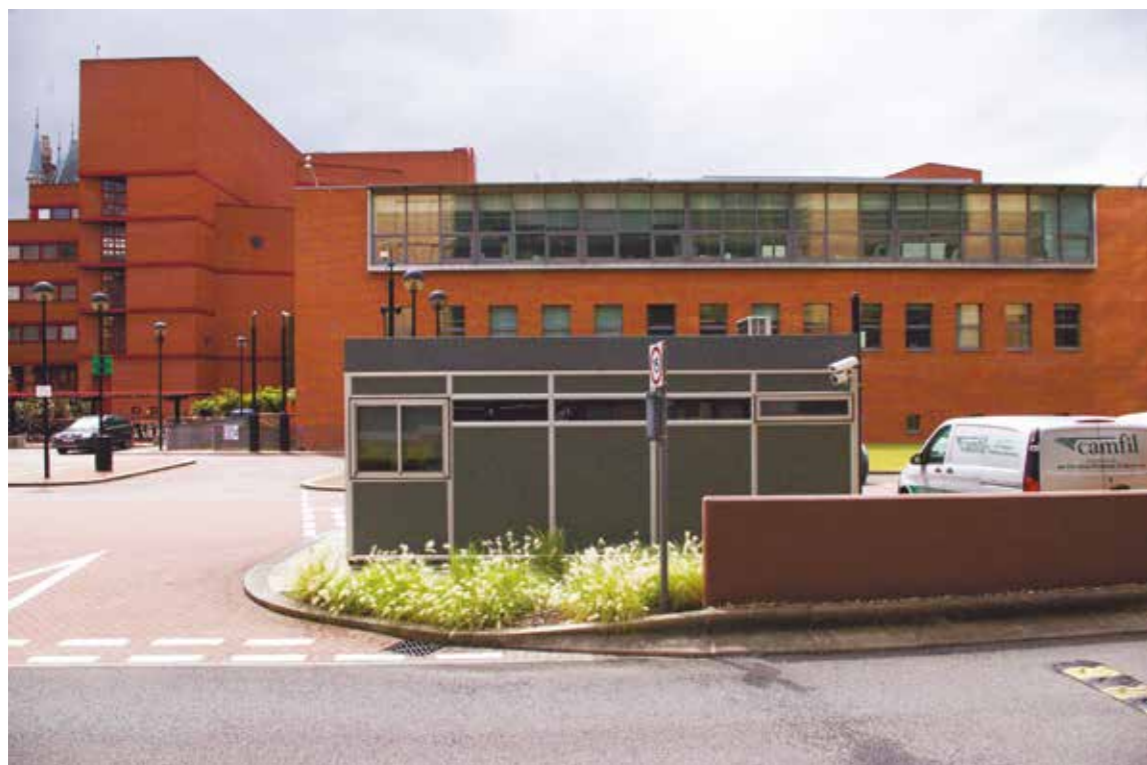
Eastern section of north elevation and Conservation Centre
