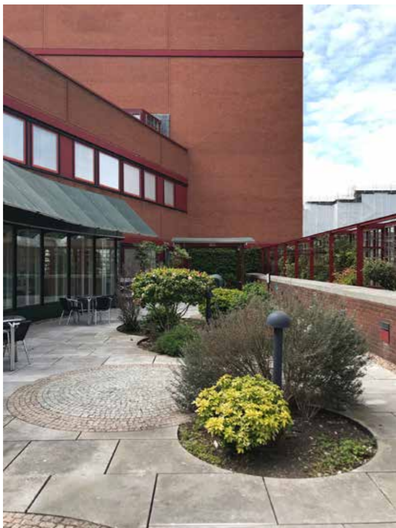
First floor terrace with former staff cafe and trellis looking west
