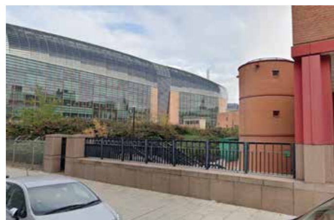
Ossulston Street external stairs and railings
