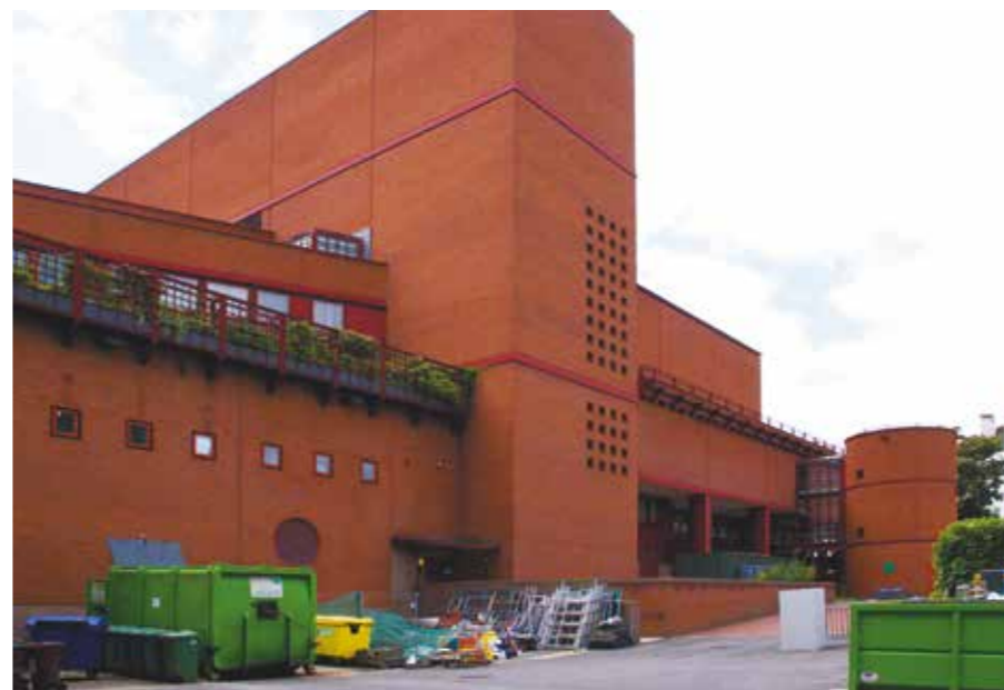
North elevation, central and eastern section with circular fire escape stair tower
