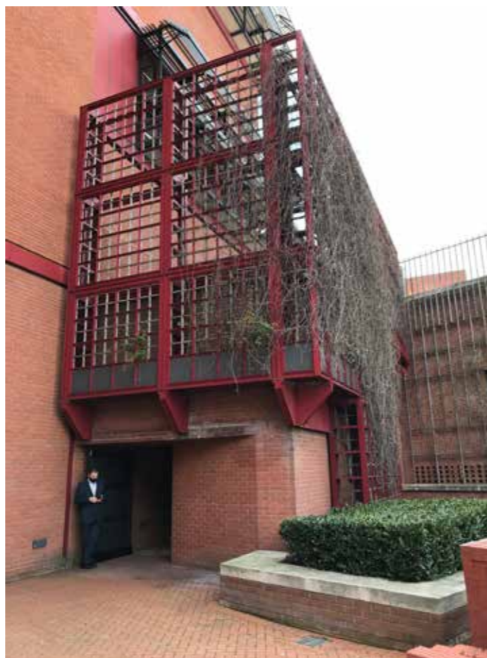
Midland Road escape staircase
