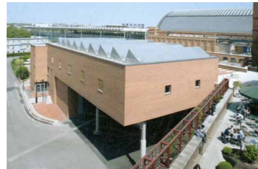
13. The BLCC from the southwest in 2007 (Architecture Today, June 2007)
