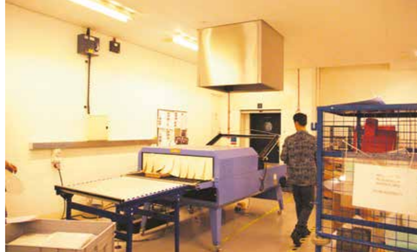
Basement 2 back wall
