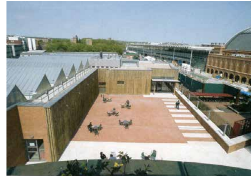
12. The BLCC from the south in 2007 (Architecture Today, June 2007)
