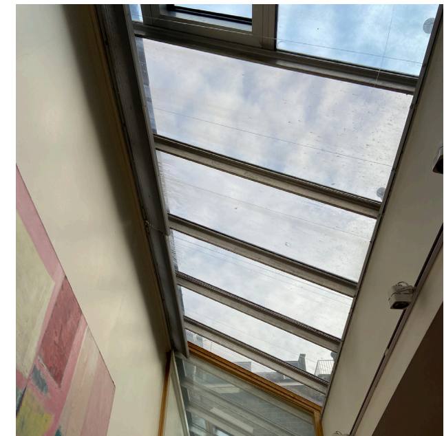
Fig. 16 Rooflight incorporated into the ground floor rear spaces
