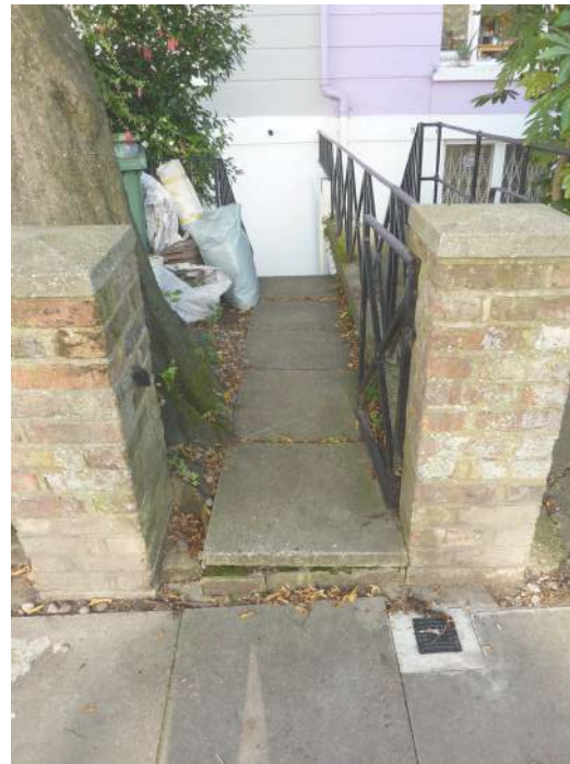
Fig.8 Uneven paving at No 10A gateposts hornbeam tree behind
