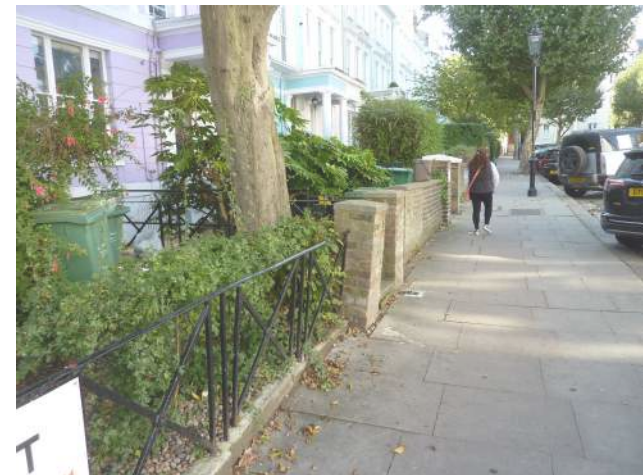
Fig.5 View of No 10A & hornbeam tree behind, pushing gatepost forward
