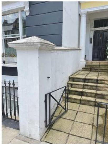
Fig.1 Gatepost and boundary wall of No 11 Chalcot Square showing capping detail
