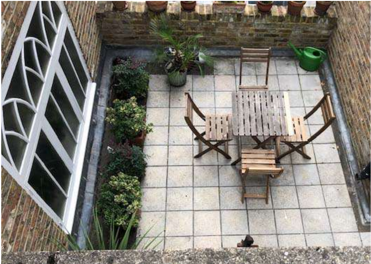
Image 08 Neighbouring rooftop at 66 Neal Street
