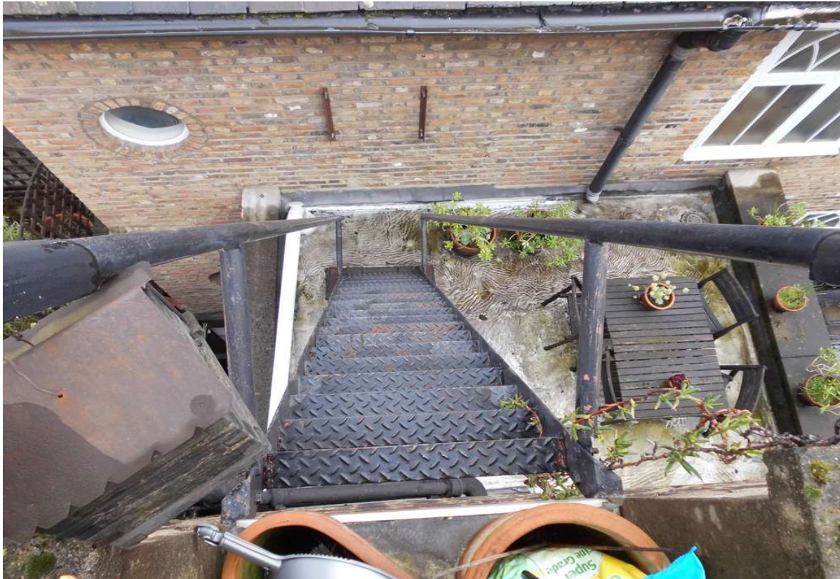
Image 06 view looking down on redundant steel stair
