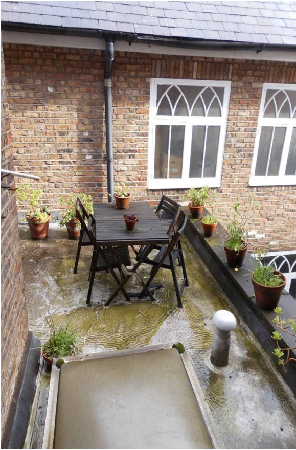
Image 05 view of existing roof
