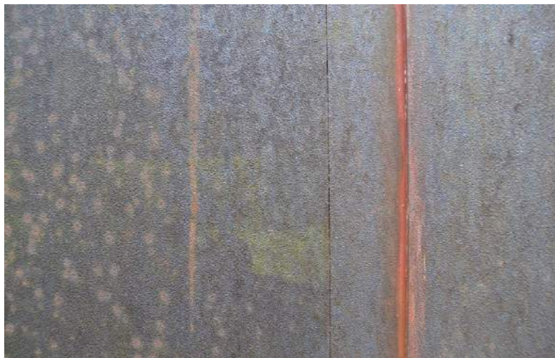
Figure 8: Close up of the oxidised surface of The Winter House
