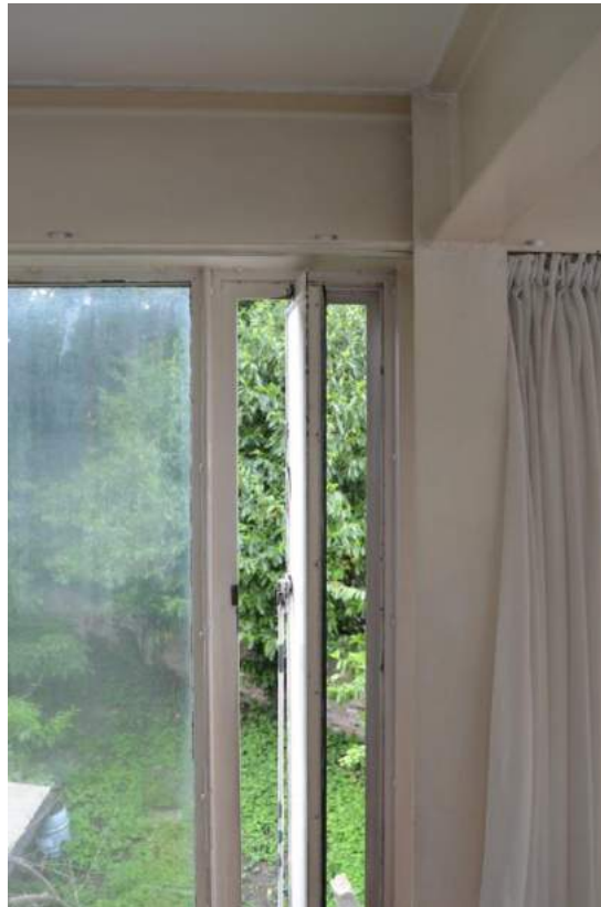
Figure 9: Shows the exposed steel beams, the 'milky hue of cataracts' on the double-glazed windows and the centre hinged vertical louvres
