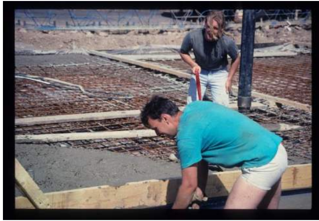
Figure 10: Laying concrete floor slabs.
