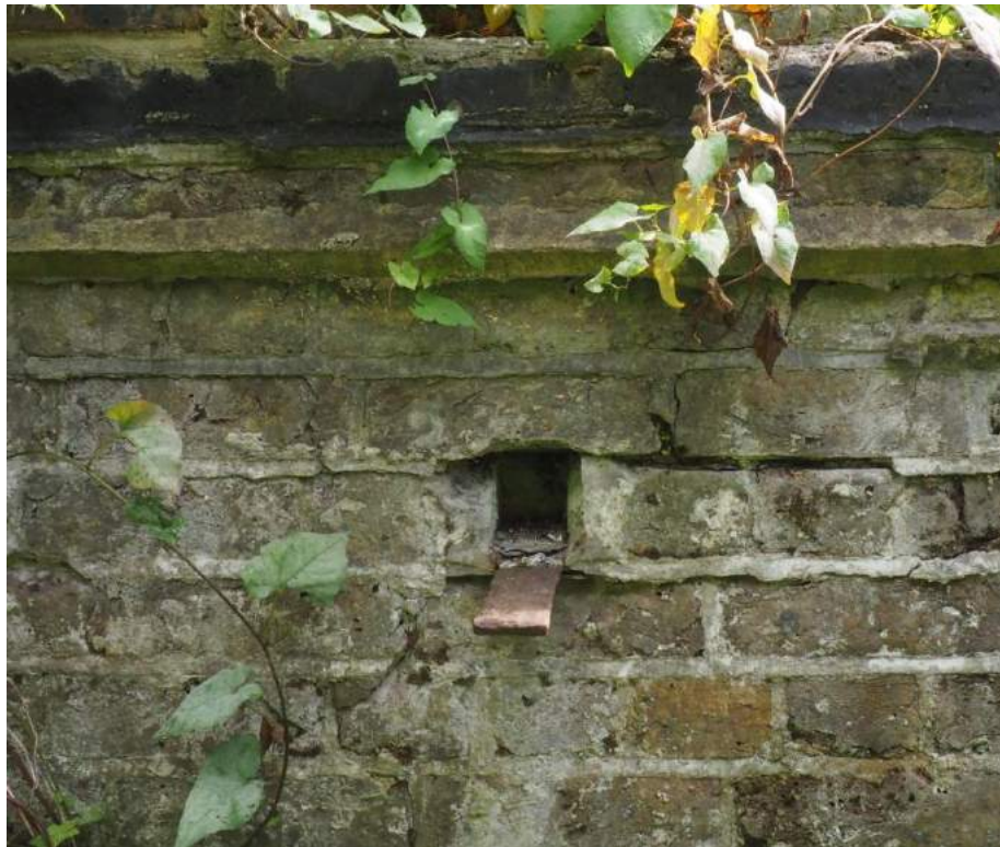
Figure 20: Close up of a cast iron fixing from the cutting which may well once have held up a glass roof.
