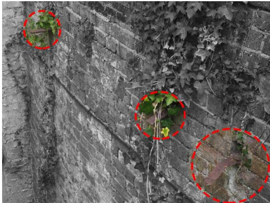
Figure 19: The cast-iron 'spandrels/bracket fixings' in the cutting, which are likely to have supported a glass roof.
