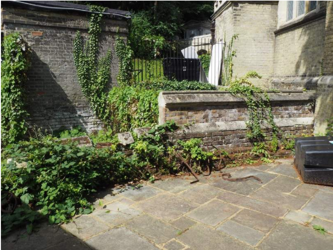
Figure 21: The surviving section of intact wall above ground, also illustrating the cutting's construction of London stock brickwork with a limestone coping.
