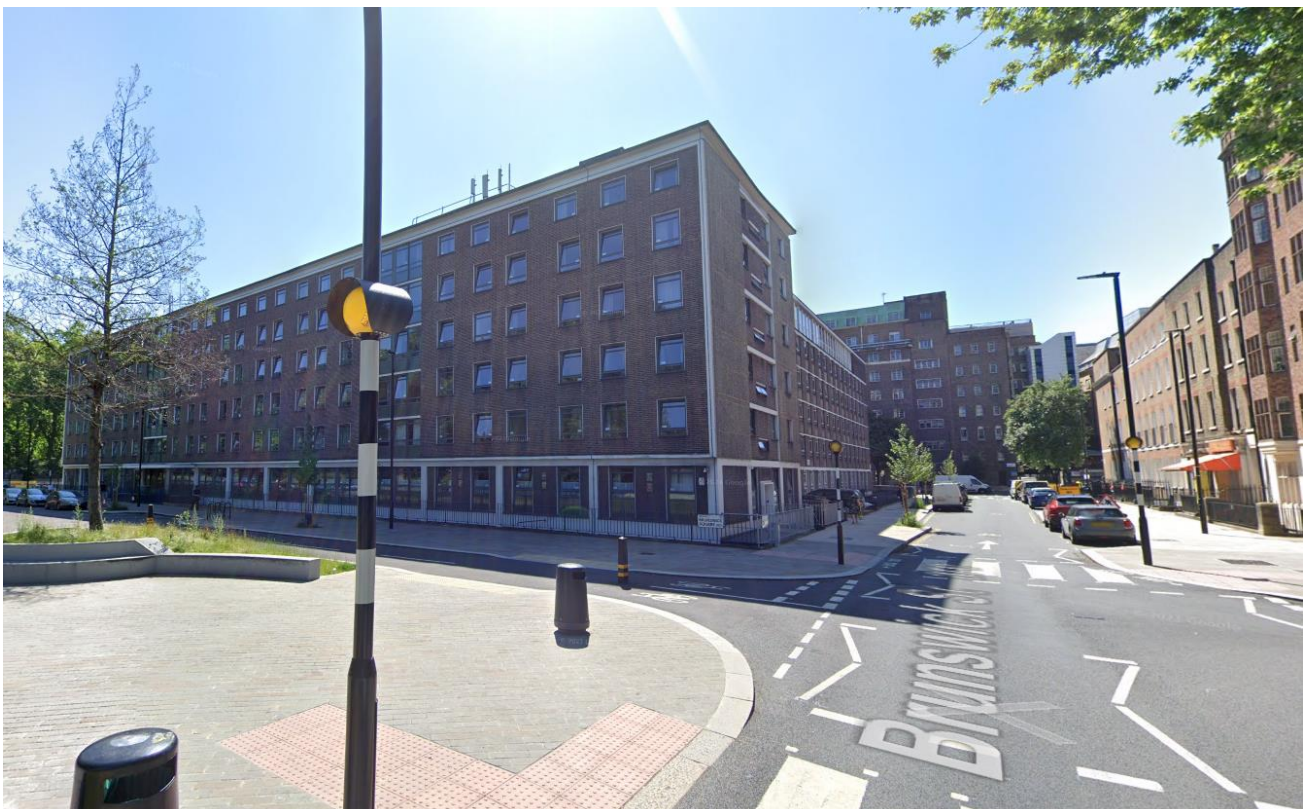
Photo 4 (below): Closer street perspective from approach from Brunswick Square
