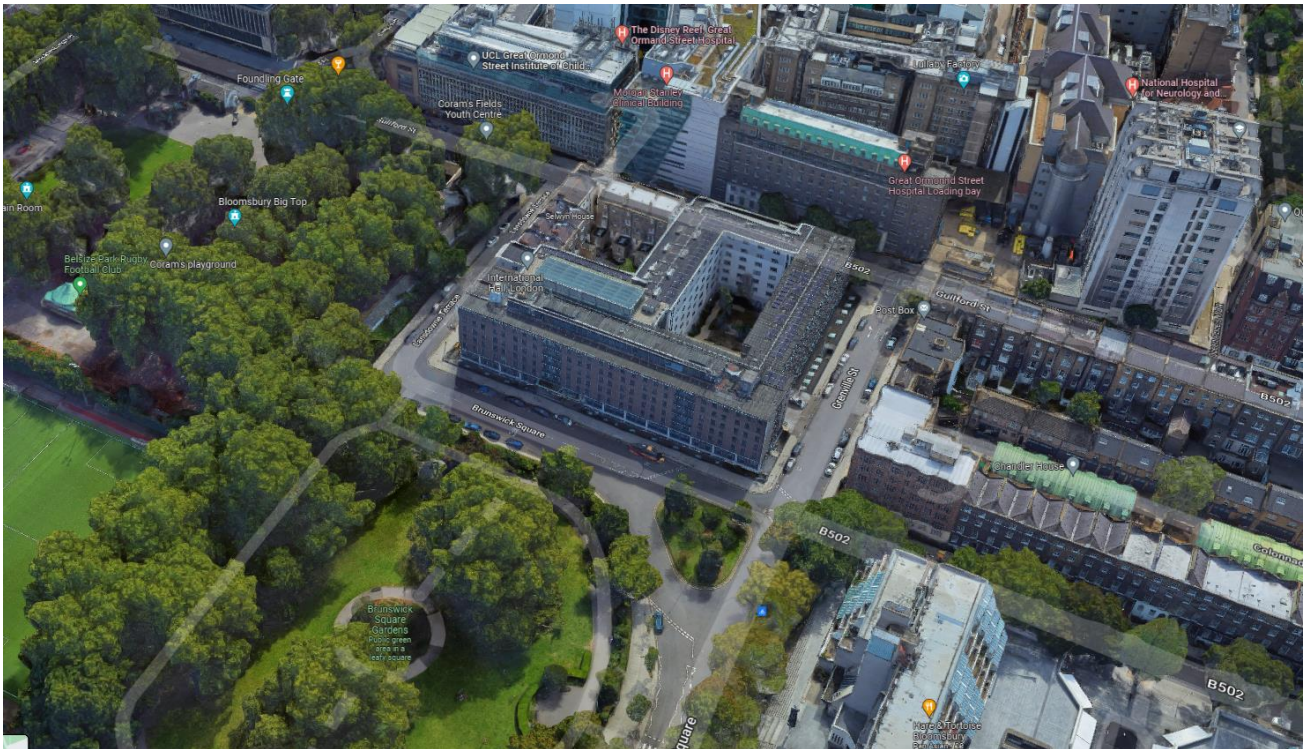
Photo 1 (below): Aerial view of main façade/roof in context
