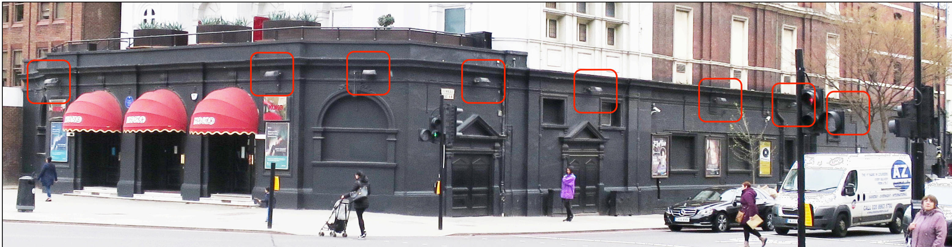
PHOTOGRAPH OF KOKO FRONT FACADE AND CROWNDALE ROAD SHOWING EXISTING FLOOD LIGHTING FIXTURES (2016). THESE FLOOD LIGHTS WERE REMOVED DURING CONSTRUCTION WORKS AND ARE TO BE RE-INSTATED IN THEIR ORIGINAL LOCATION.
