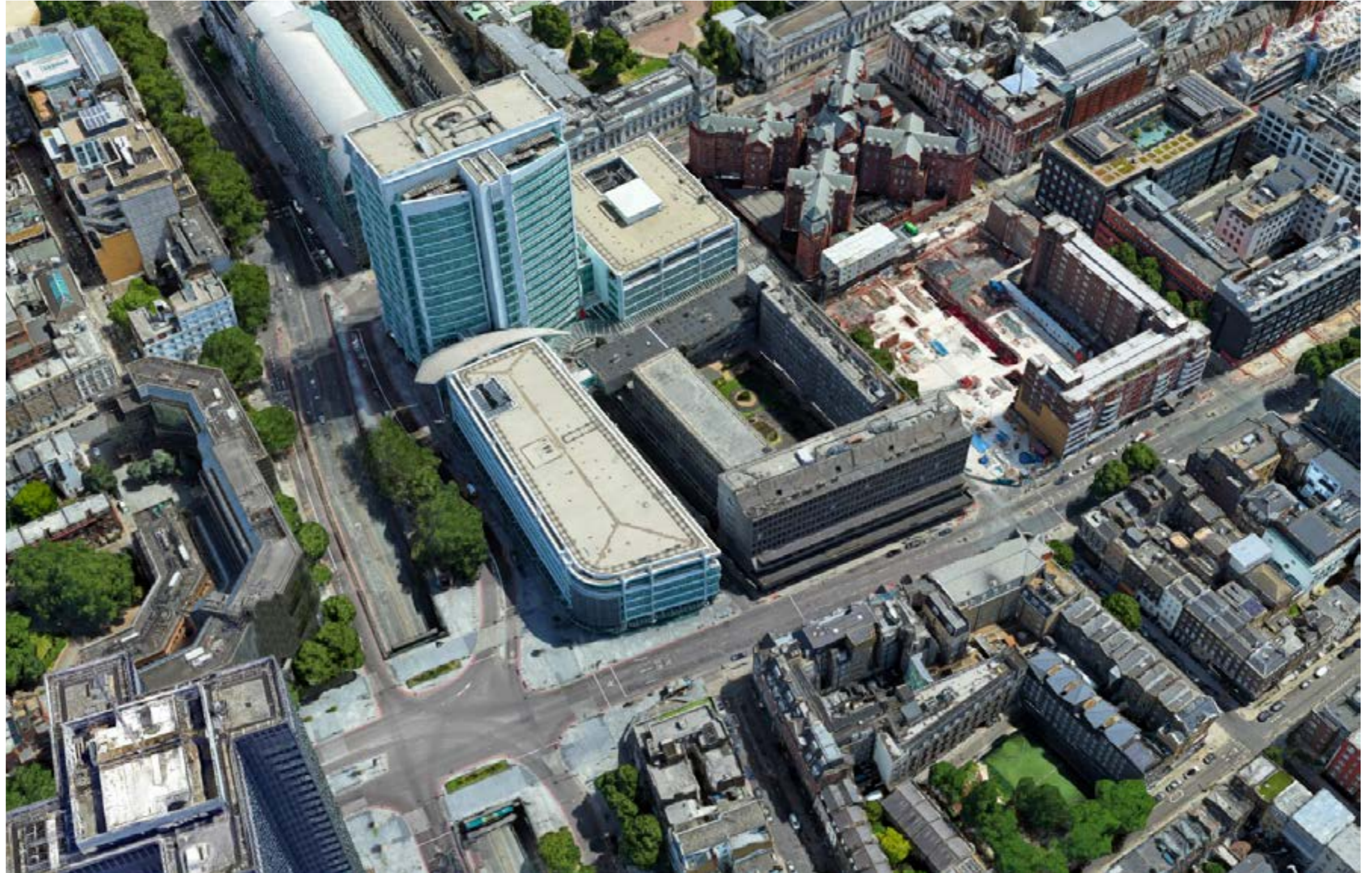
Overview of existing building from the west
