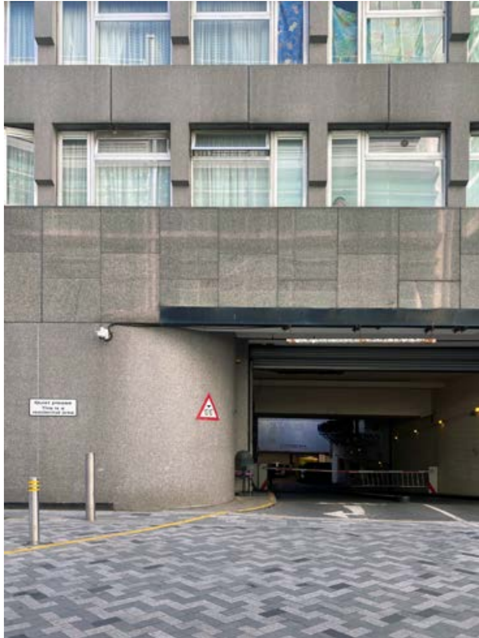
View of car park entrance from Beaumont Place
