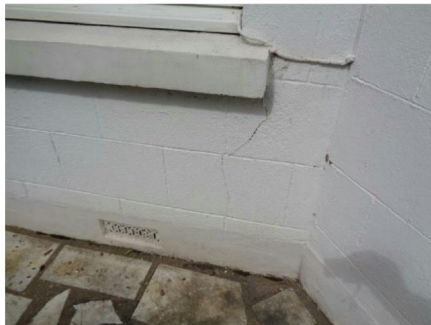
Cracking to the right side of the front bay
