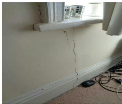
Cracking beneath the front window in flat 3
