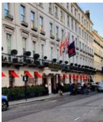
BROWN'S HOTEL, ALBEMARLE STREET W1, CONTEMPORARY VIEW
