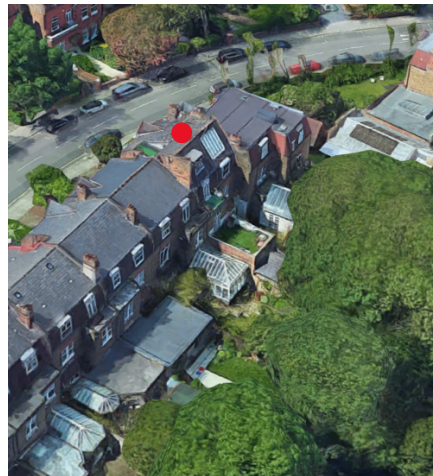
Figure 2.2 – Rear of Property.
