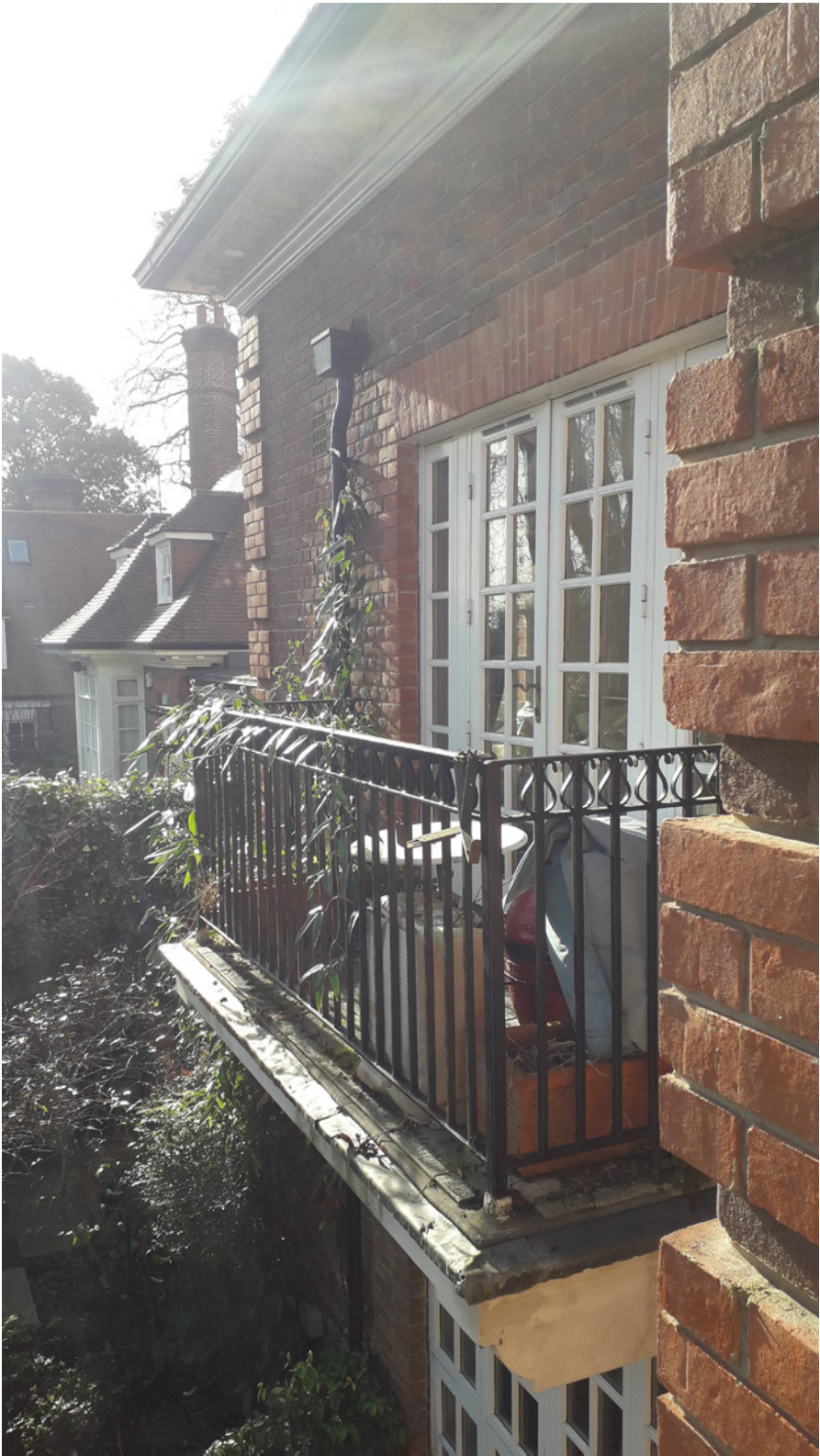
Metal balustrades to be replicated for other two balconies
