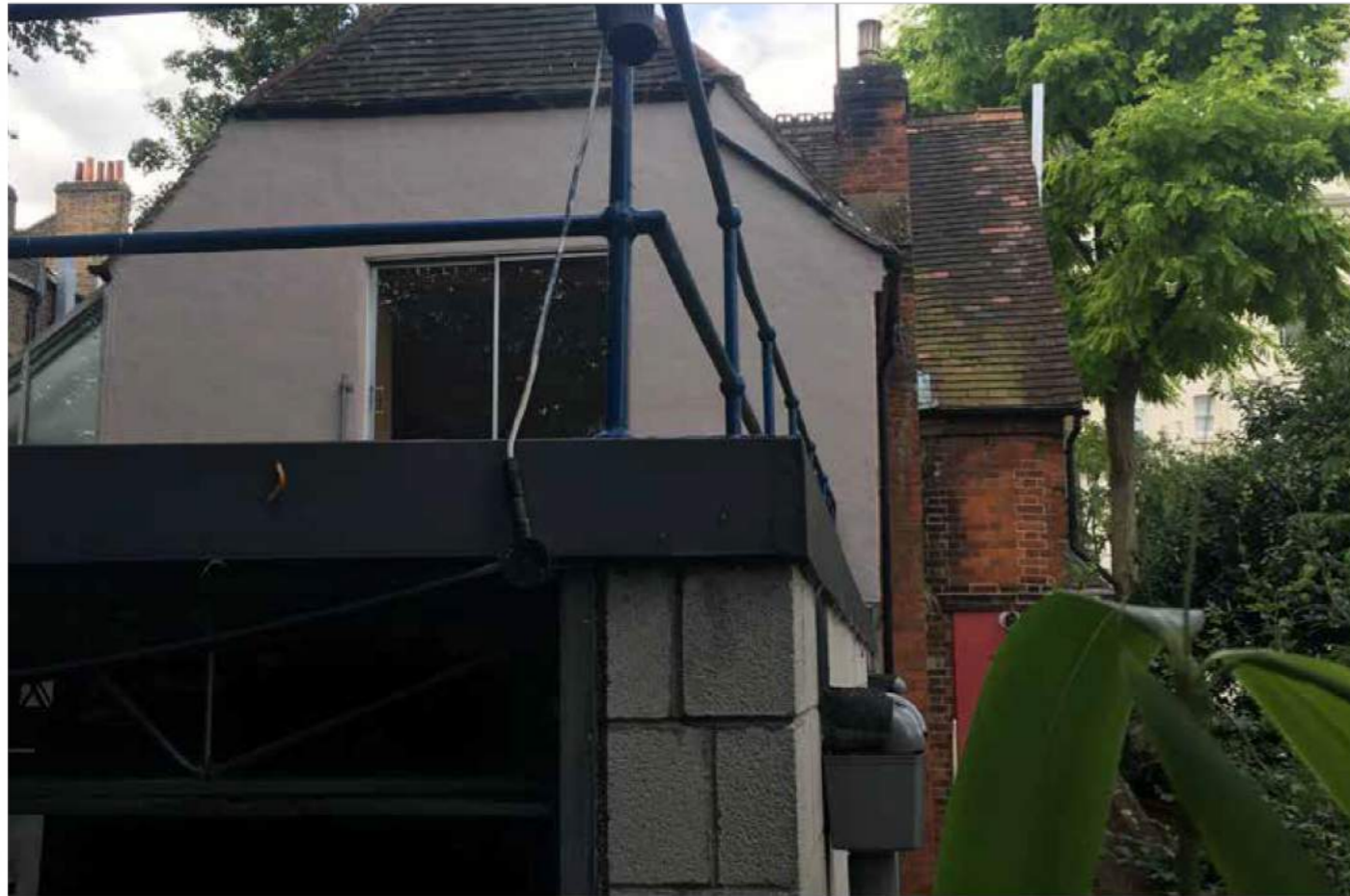
Existing view from north-east corner of the rear garden
