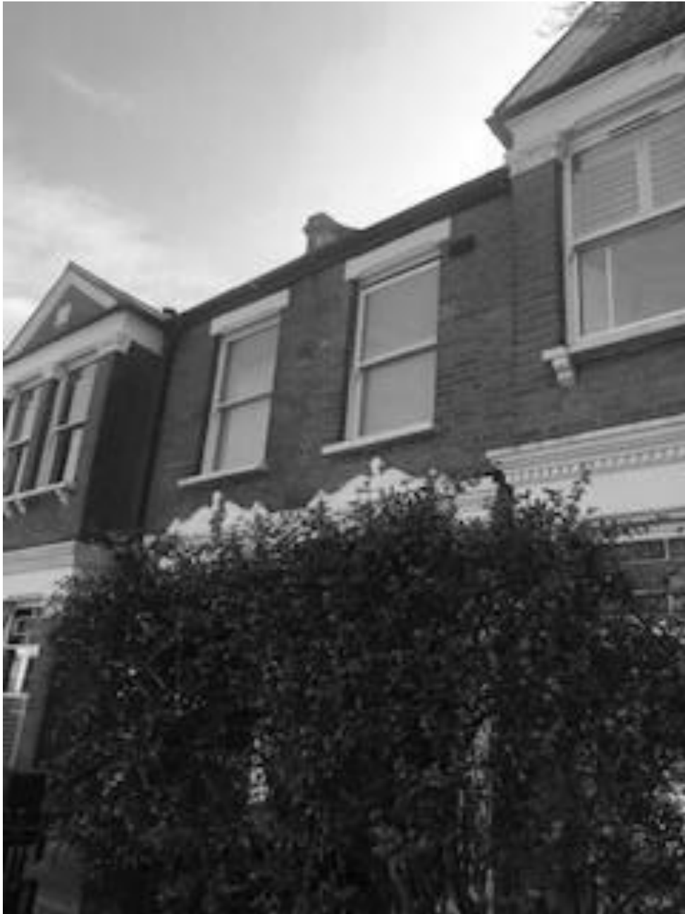
7. View of parapet wall at no.26/28 junction
