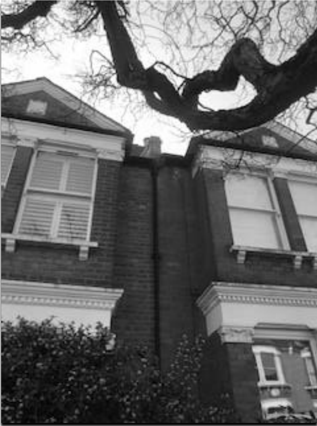
6. View of parapet wall at no.24/26 junction
