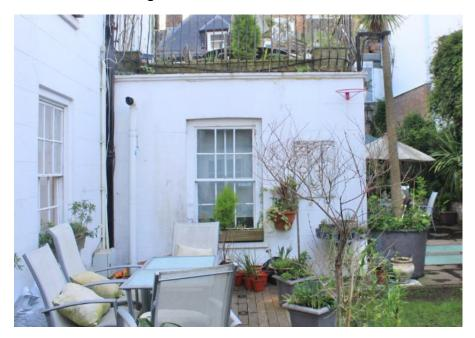
The window, shown above, will be removed along with materials below to form a new opening from the reception room into the proposed orangery.
