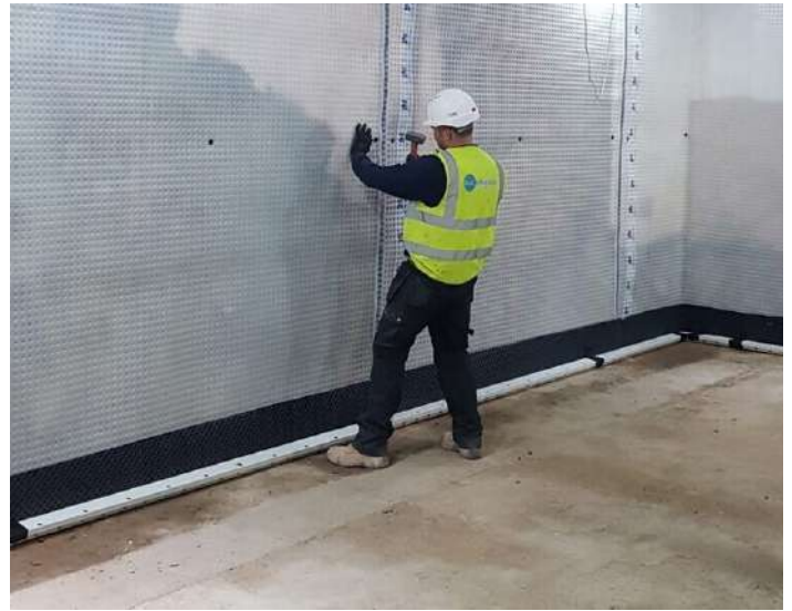
Example of a standard Type C cavity drain
