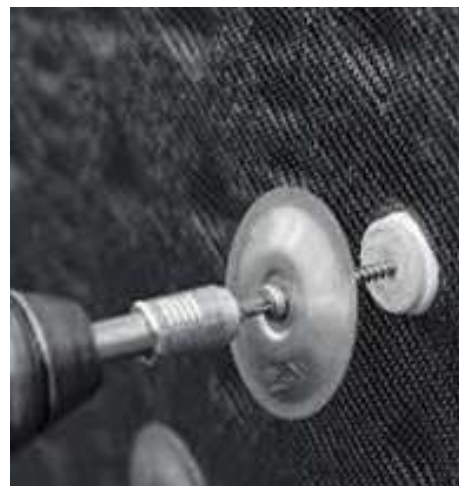
Example of fixing for fire resistant membrane
