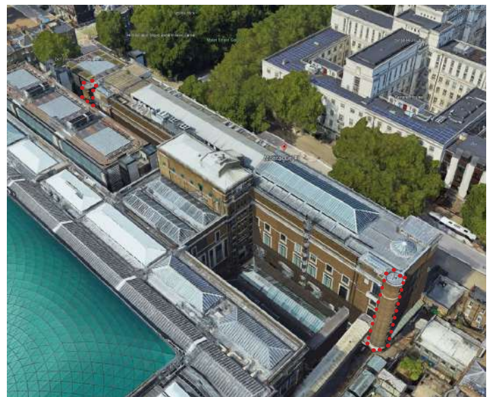
Aerial view of south east elevation of the KEB showing the stair turrets that access the basement tunnels
