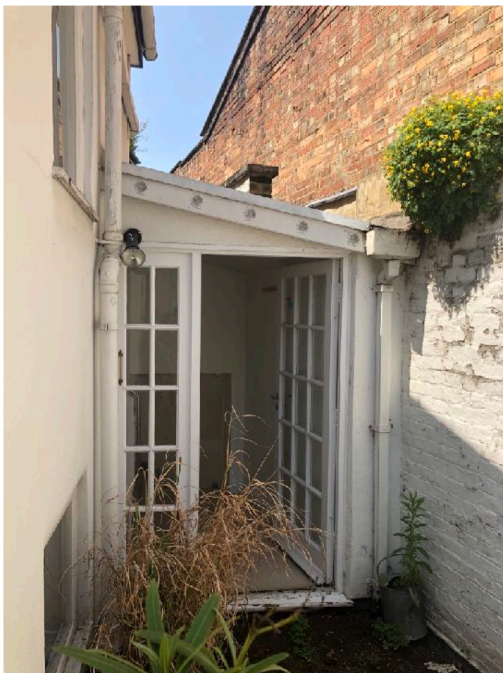
view of rear addition
