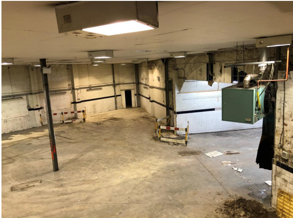
General view of secondary warehouse area (zone 4).
