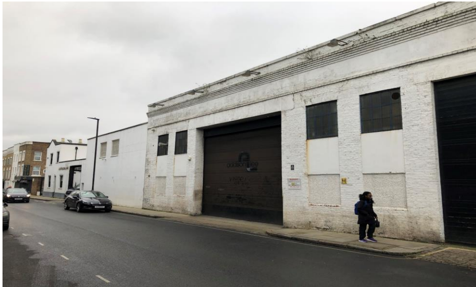
General view of existing elevation showcasing begrimed painted masonry and spalling areas of render.
