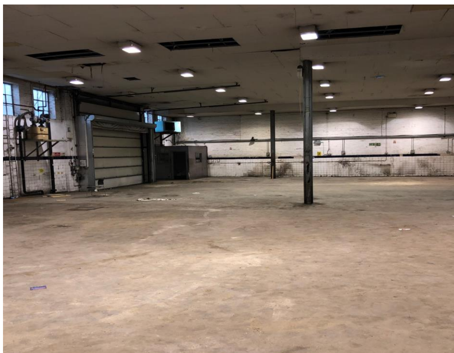
General view of primary warehouse area (zone 1).
