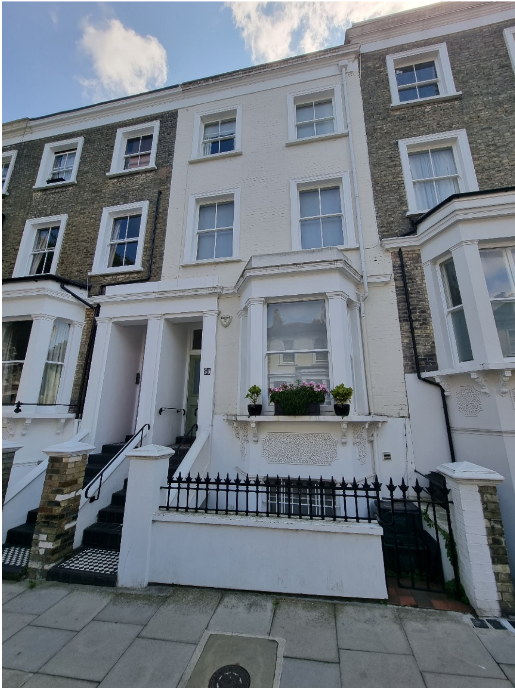
Figure 2 - Photograph of the existing front facade
