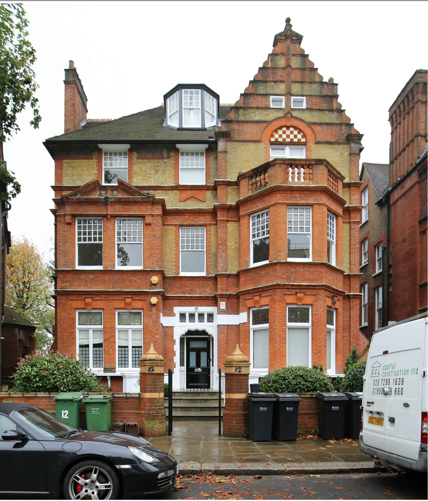
PHOTO OF EXISTING FRONT ELEVATION
