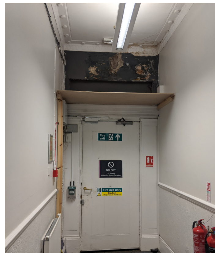
Image of damage caused to interior of front door at ground floor level due to water ingress to level 01 balconies - Proposal is to repair balconies and damage to entrance doors.
