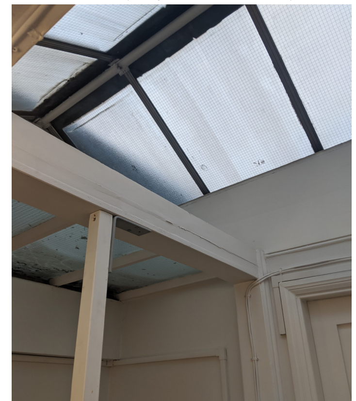
Image of a rooflight to level 04 and insertions to capture ingress of water - Proposal is to replace rooflights to address water ingress and prevent ongoing damage to building fabric
