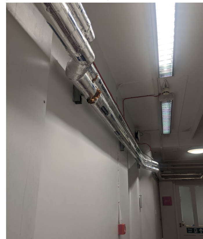
Example of exposed electrical and mechanical services that occur throughout the building - Proposal is for replacement services to be rationalised and consolidated lessening their prominence and improving their appearance
