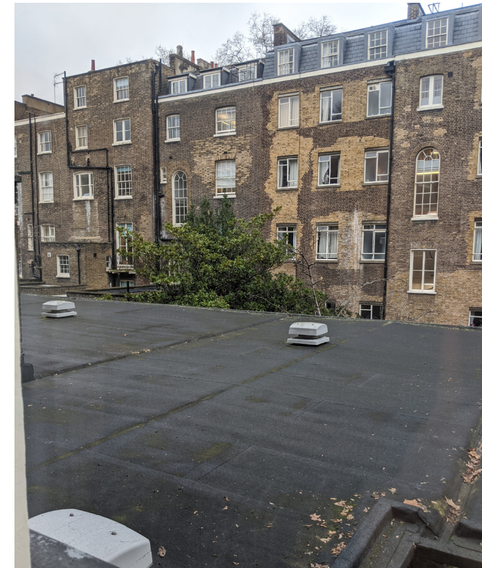
Existing rear flat roof - Proposal is to refurbish flat roof to improve thermal performance and address historic design issues resulting in water ingress. Edge protection to be added to provide safe access
