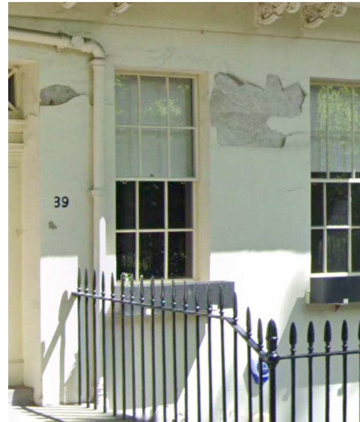
Damaged stucco to Gordon Square elevation - Proposal is to repair and redecorate Stucco to ground floor and basement levels
