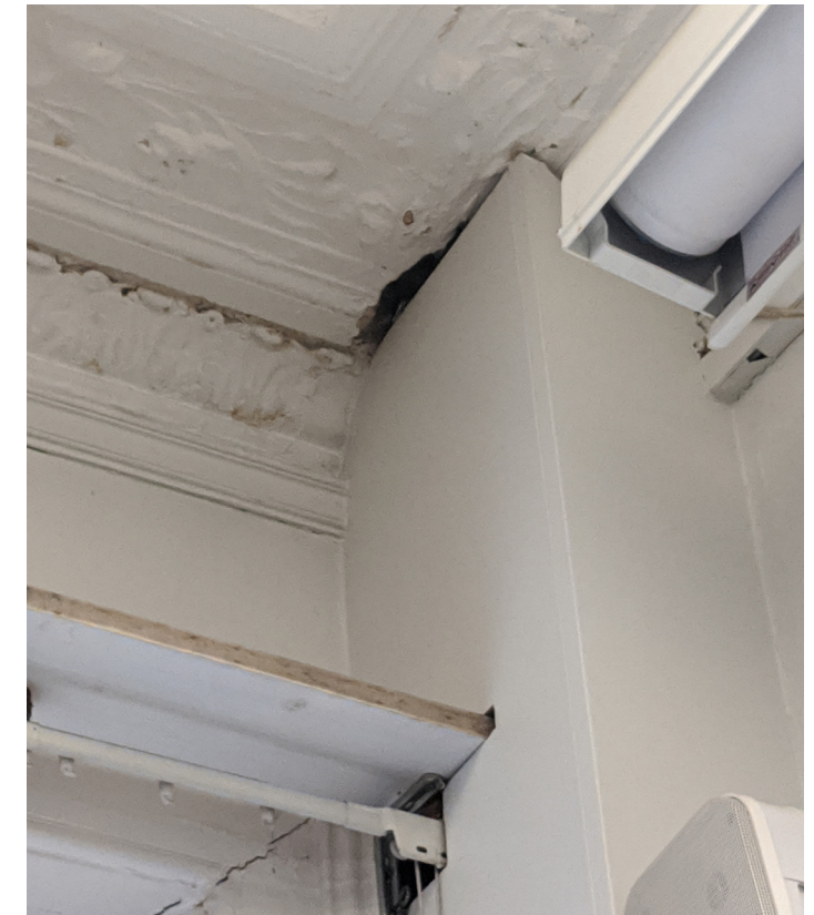
Example of existing service boxing clashing with historic detailing - Proposal is to consolidate service risers and remove them from primary rooms to front of terraces. Poor quality enclosures to be replaced
