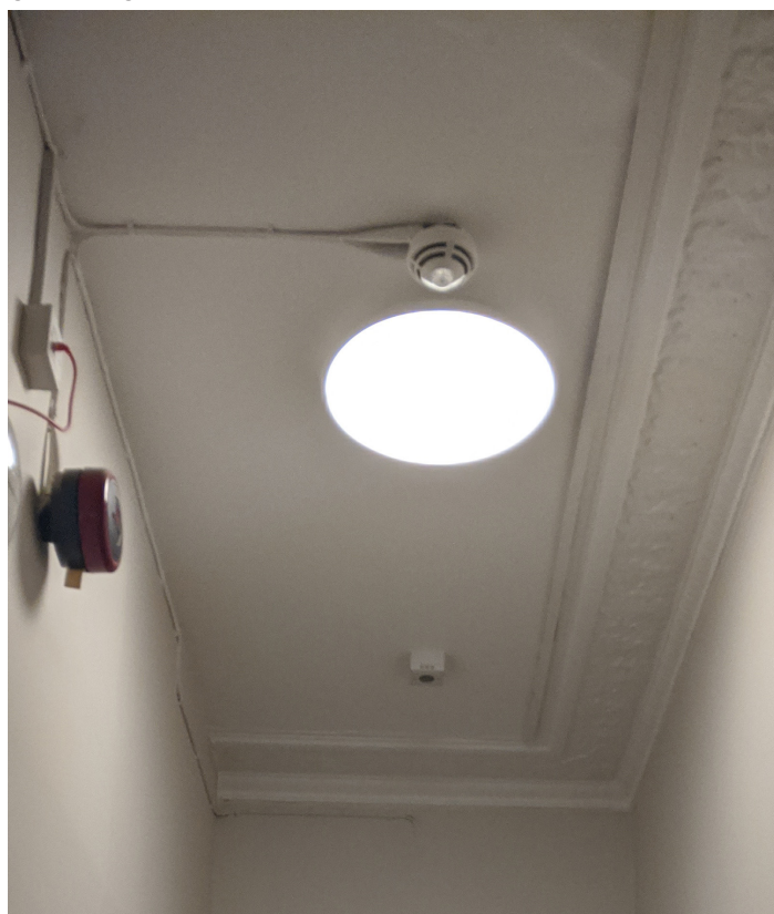
Example of existing corridor partition that has cut through original cornicing and exposed electrical services - Proposal is to remove a number corridor walls that bisect historic rooms and address unsightly services.
