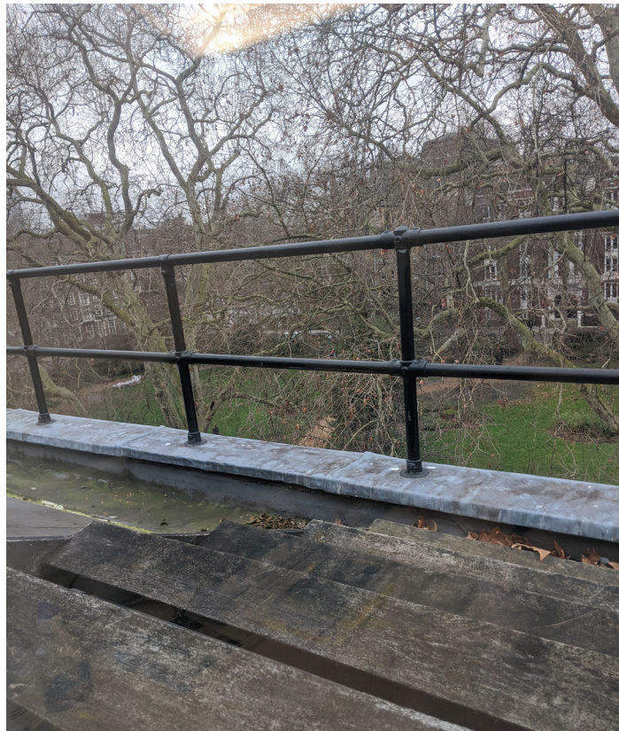
Existing timber steps to level 04 roof and existing roof guarding system - Proposal is to improve appearance and safe access to roofs by replacing steps and guarding.
