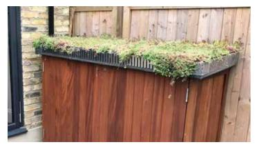
All the elements required for a successful green roof have been designed into the M-Tray® modules at our UK nursery to ensure strong, healthy long-lasting vegetation. The trays are grown on site for at least 6 months and all will have been through at least one Spring growing season; so the plants are well established, healthy and strong, and fully integrated into the substrate (unlike sedum blankets, which are not).
