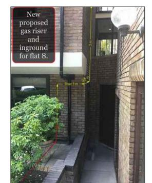
PLATE 1: PROPOSED GAS PIPEWORK CONTINUES THROUGH RECESSED AREA BETWEEN NORTHERN AND SOUTHERN BLOCKS OF FLATS. FOR REFERENCE, SEE PLATE 1 ABOVE.
