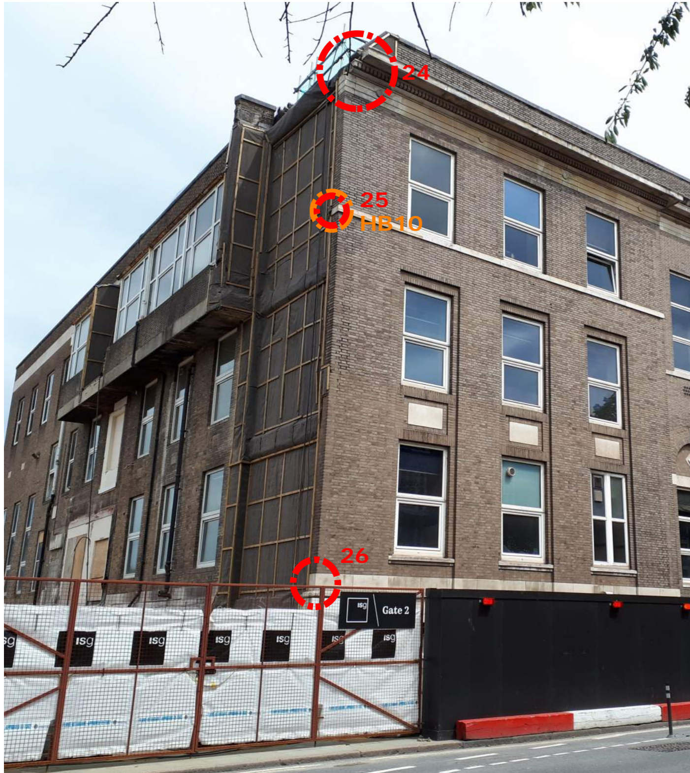
EDC NORTHWEST CORNER ELEVATION
