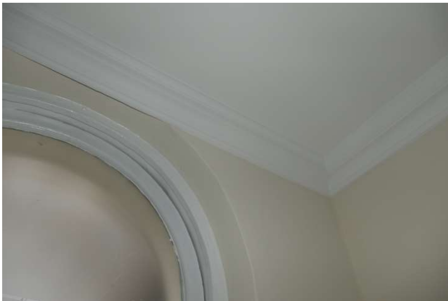
Photo 16: The modern cornice that crudely overlaps the windows heads within the rear outbuilding.
