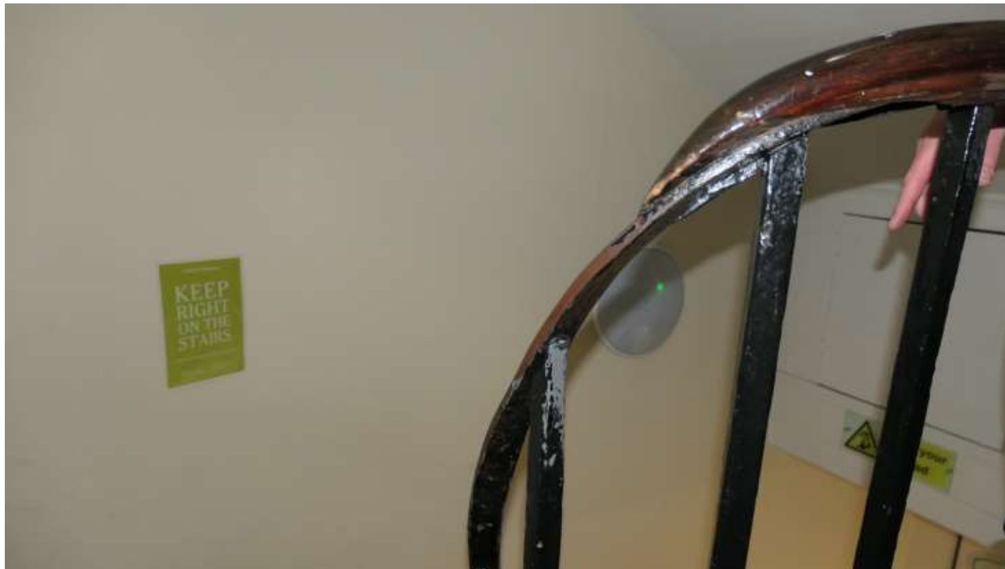
Photo 10: A crude truncation of the handrail to the basement.
