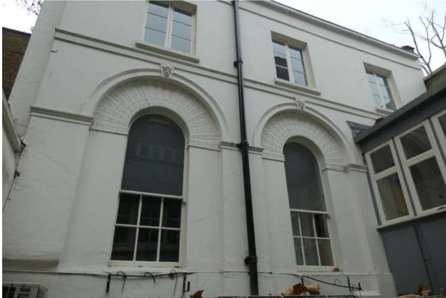
Photo 4: The arched windows to the rear outbuilding with Coade dressings.
