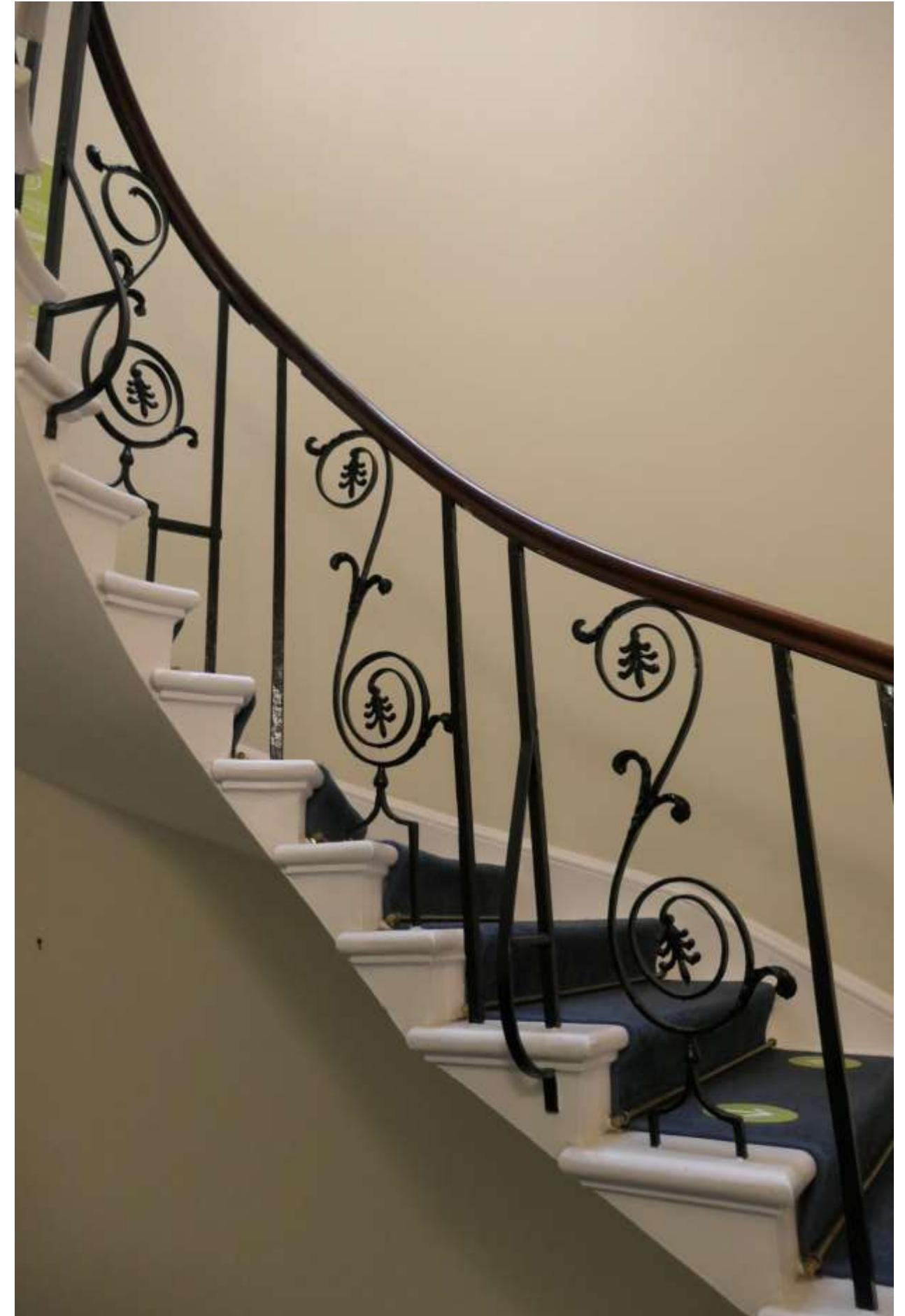
Photo 9: A detail of the cantilevered stone staircase with fine wrought S-scroll balustrade.
