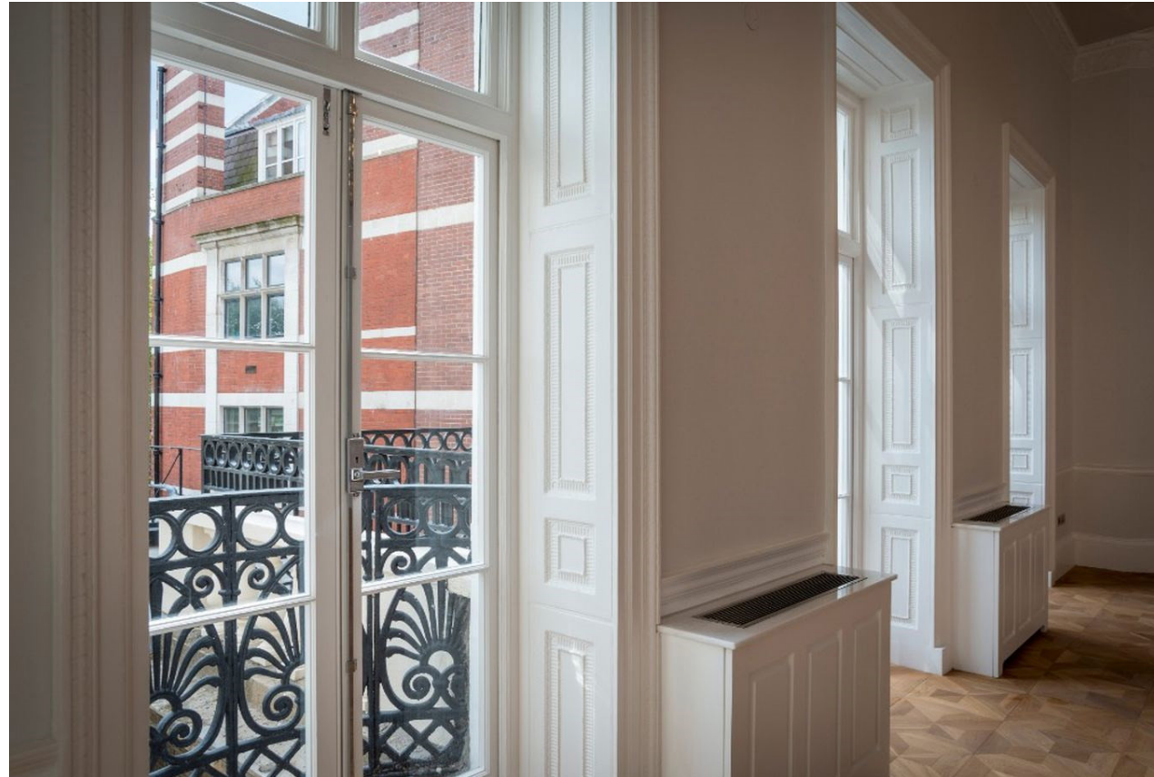
Example of wall-mounted fan-coil units concealed with timber-panelled casings
