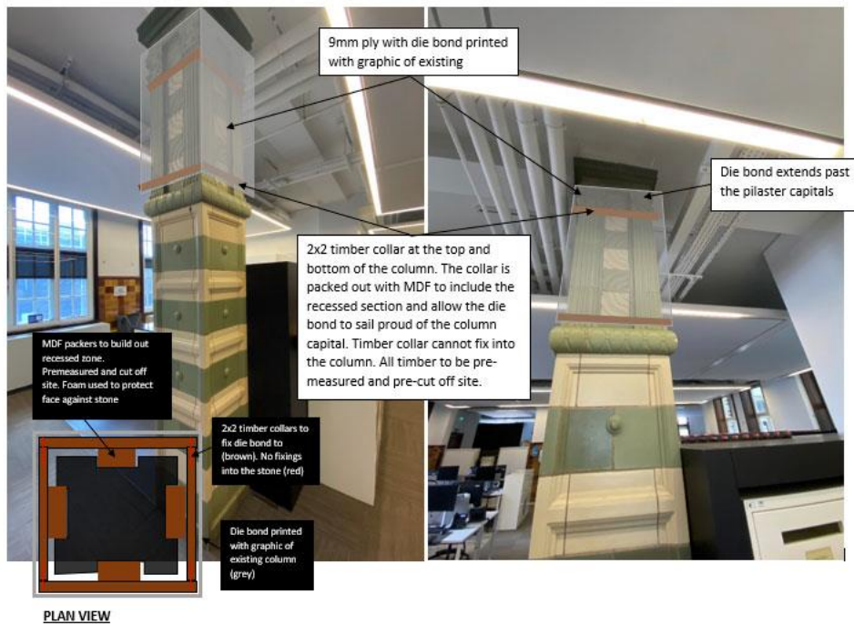
Figure 4 - encapsulation hoarding to the column
