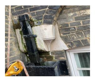
Buddleia removed. Hopper head and cast-iron work to be repaired as well as cleaning brick and stonework.
