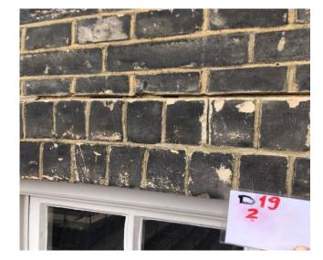
Tidying of bed mortar joints to brickwork to be cleaned and repointed
