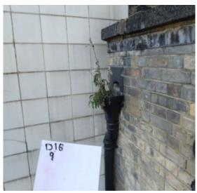
Buddleia growth in hopper head to be removed and cast-iron work to be repaired as well as cleaning brick and stonework.
