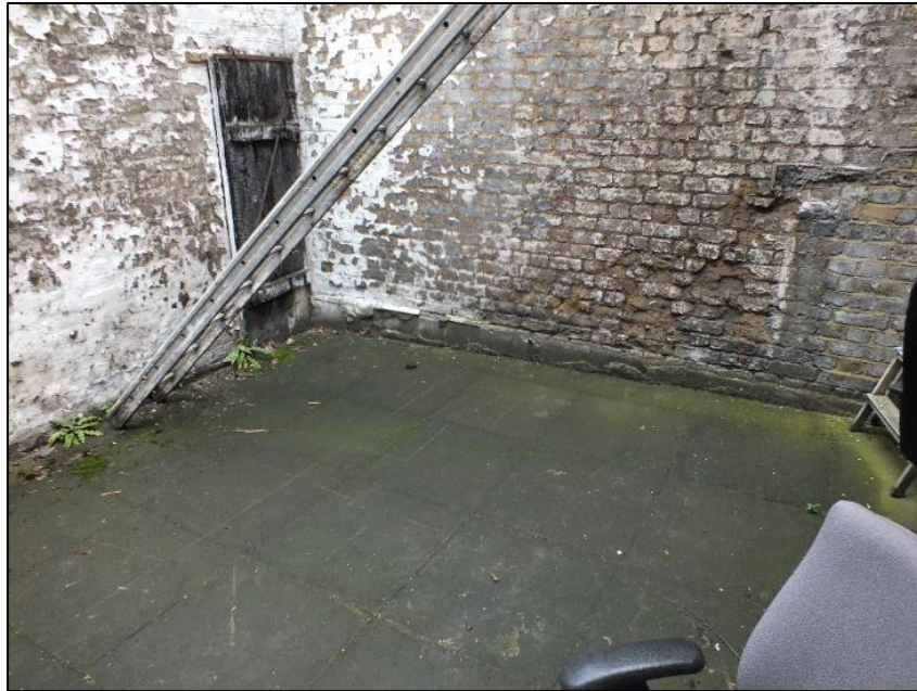
Photo 3: Yard area to the rear of No. 110, looking west
