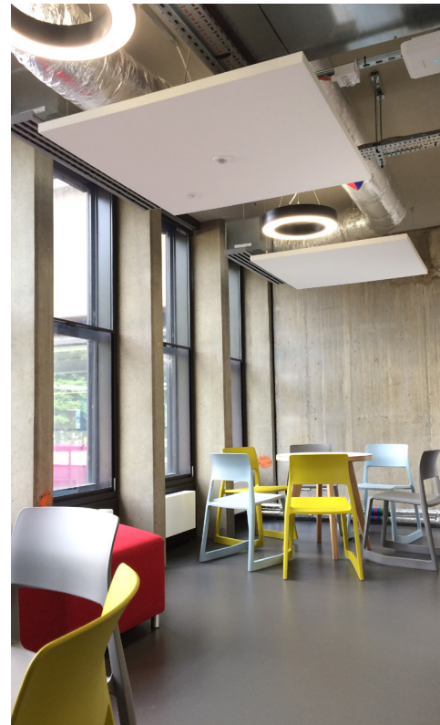
Breakout space - exposed soffits and acoustic rafts - new secondary glazing to existing facade to Phase 1, Level 4
