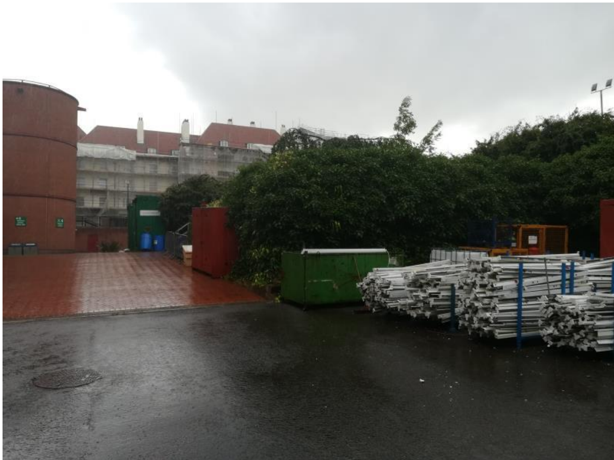
Photo 4: Looking north-west into the western half of the Site, showing the southern half of G12 (centre) as a point of reference.
