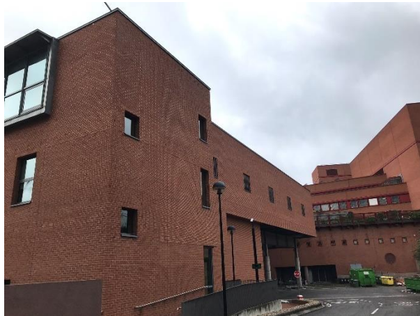
Photograph 8: main building within Development Site
