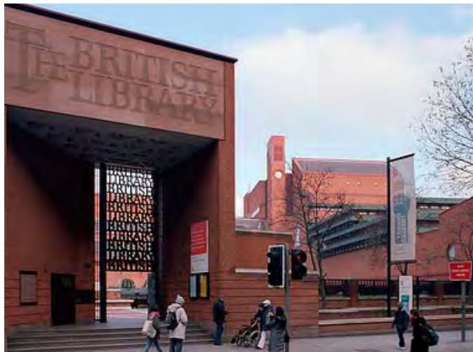
5 Euston Road Main Entrance
