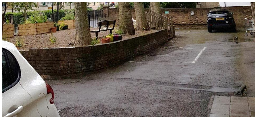
Photo 1 – tarmac to be retained and tested for strength for ground protection for roots below.
