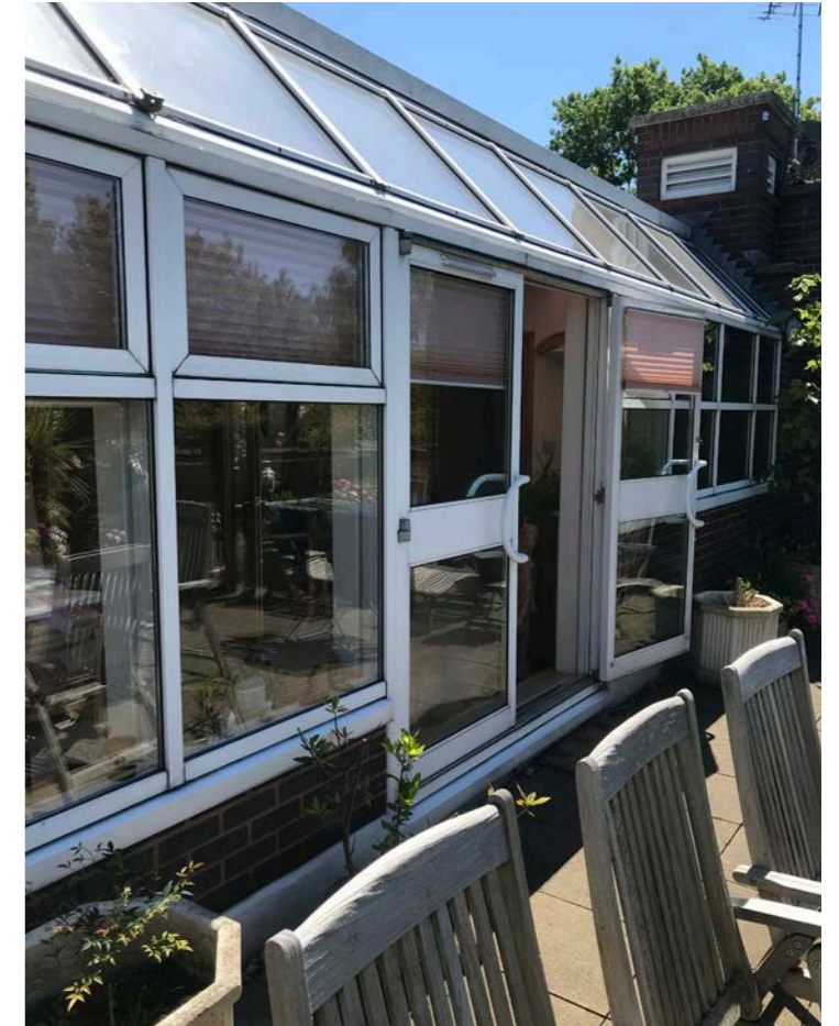
Existing Rooftop Extension
