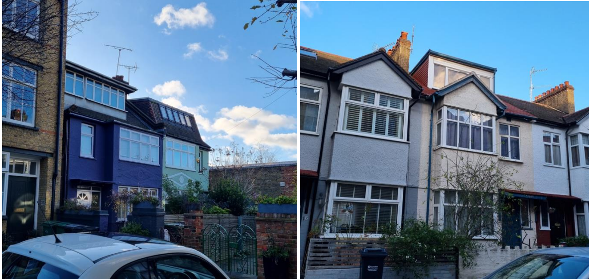
Figure 3 - No 19 (P9601467) and No 21 (2010/0962/P) and No 15 Leighton Place
