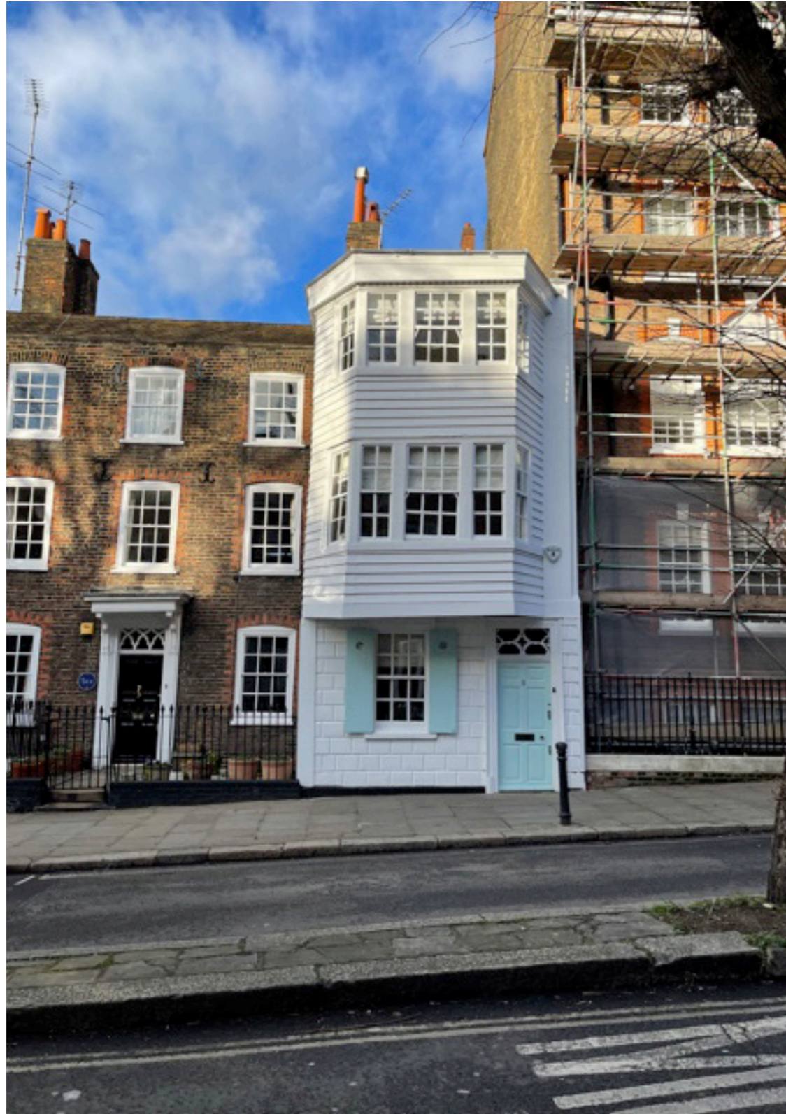
Precedent of traditional painted timber weatherboarding used on an elevation of a property in Hampstead
