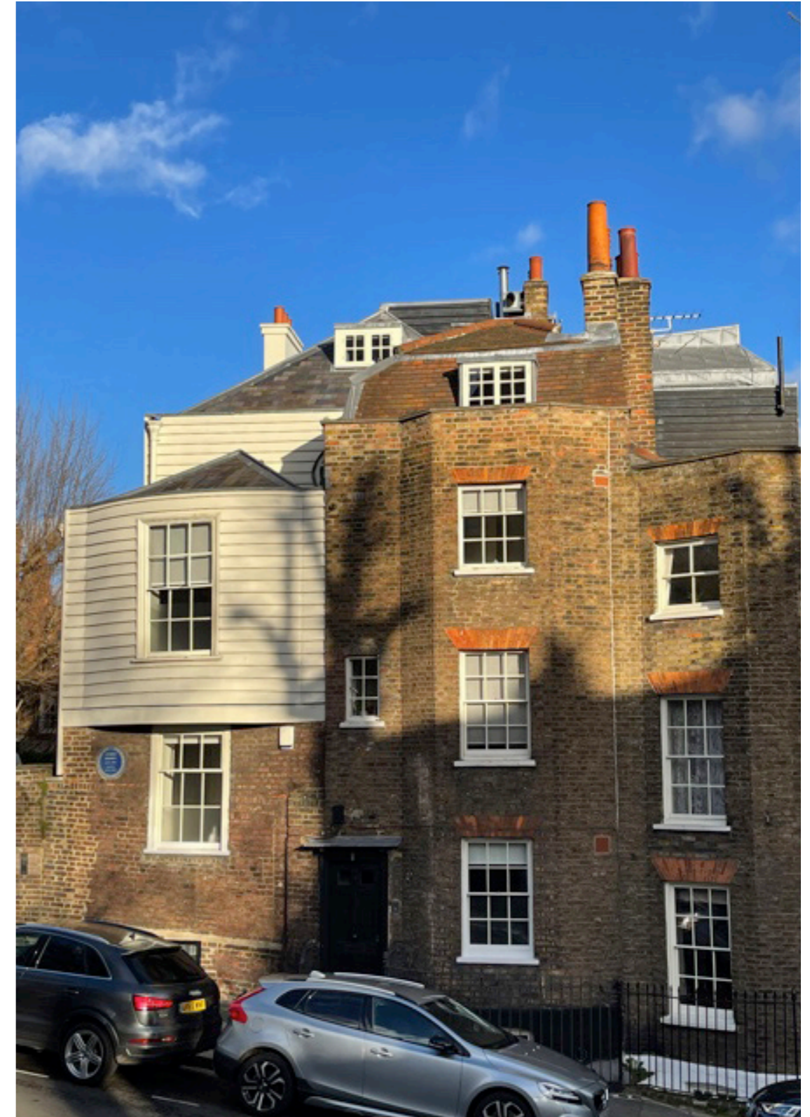
Precedent of traditional timber weatherboarding used at Romney's House, 5 Holly Bush Hill, Hampstead. As per granted applications 2010/3809/L, 2010/0943/L and 2009/2026/L.
