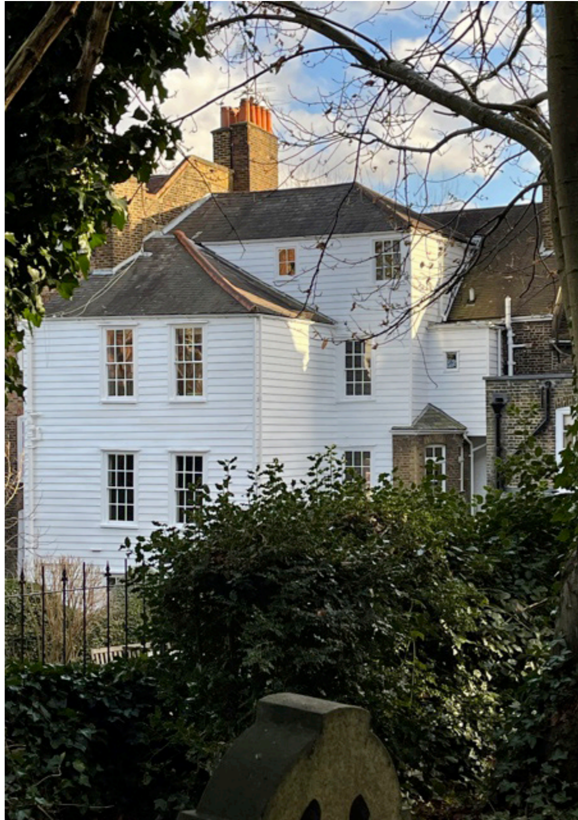
Precedent of traditional painted timber weatherboarding used at Number 10 Church Row, Hampstead.
