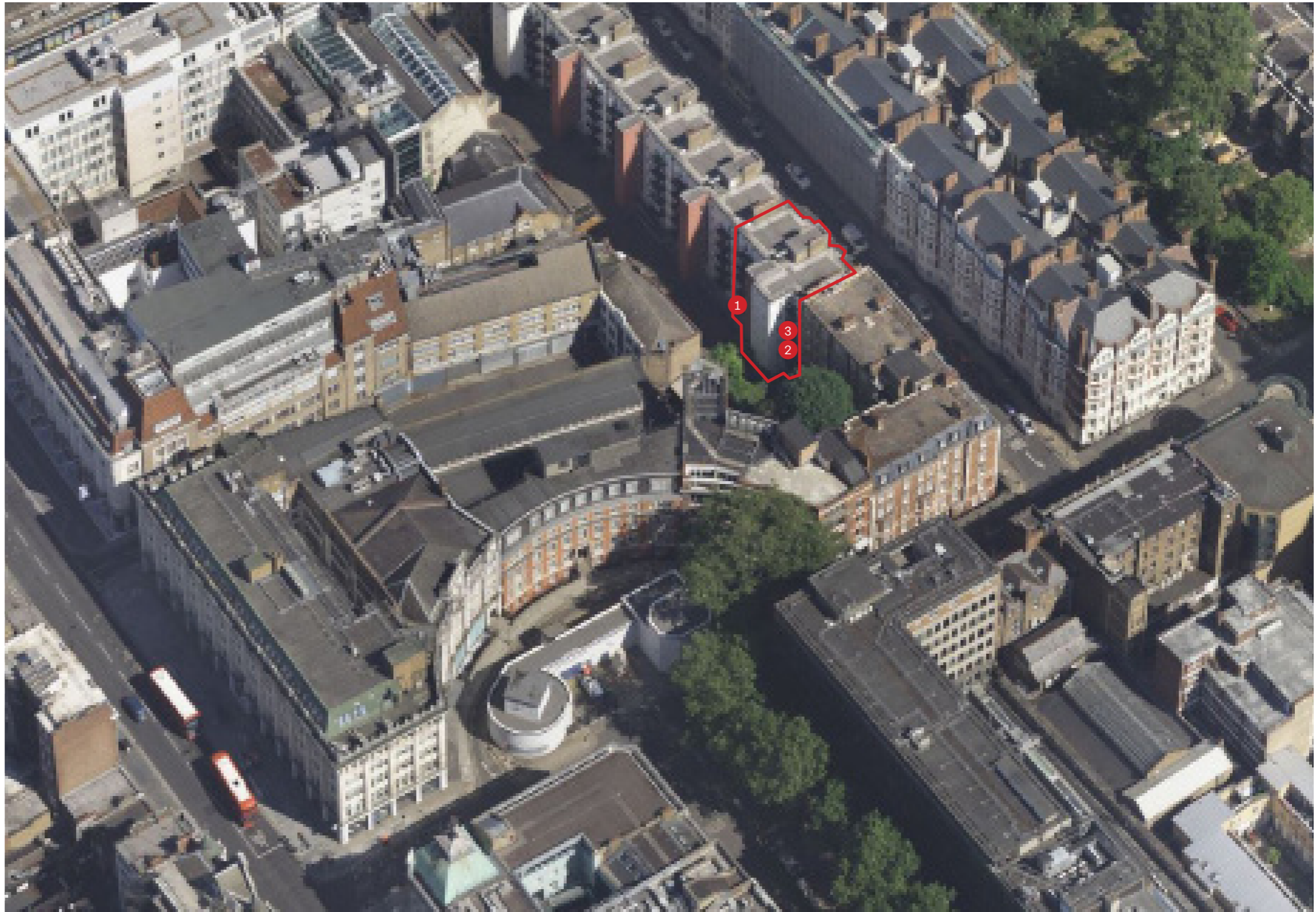
Aerial view of North Crescent
