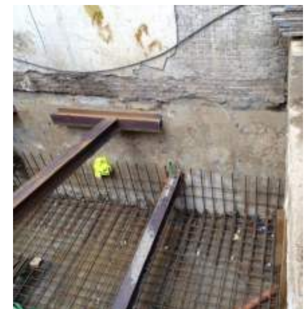
Figure 5 – Typical temporary propping
