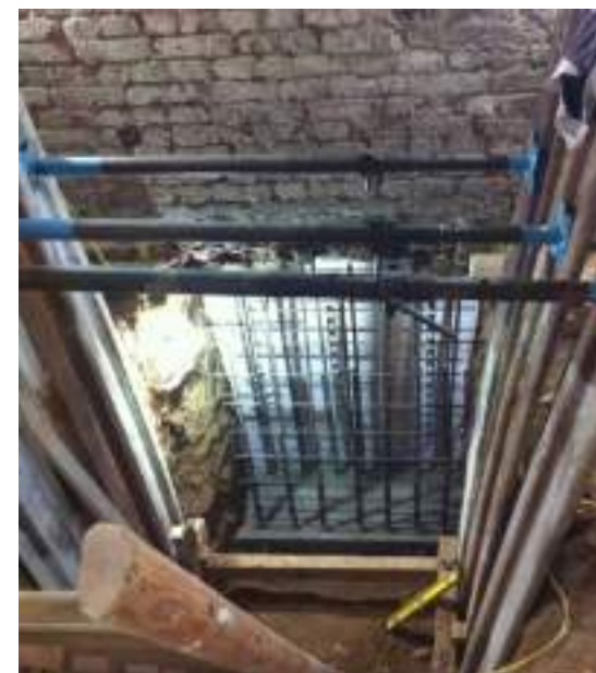
Figure 4 – Typical underpinning bay
