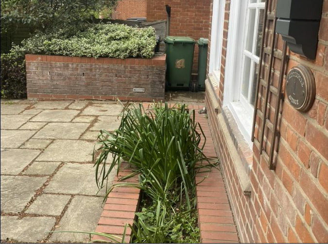
Existing concrete block paving and binstores
