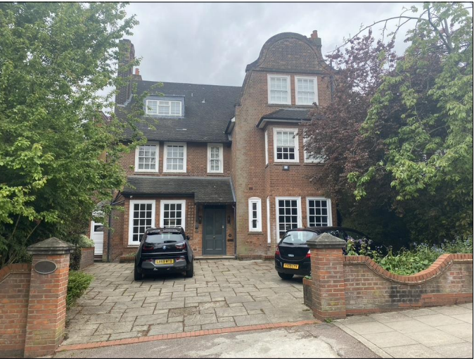
Existing boundary walls and entrance, both trees to the right now not existing. Purple cherry blew down July 2021 and second cherry was removed by tree care in 2011.
