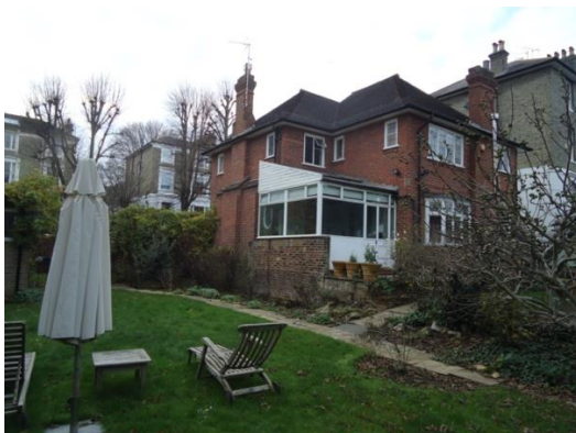
South elevation and conservatory
