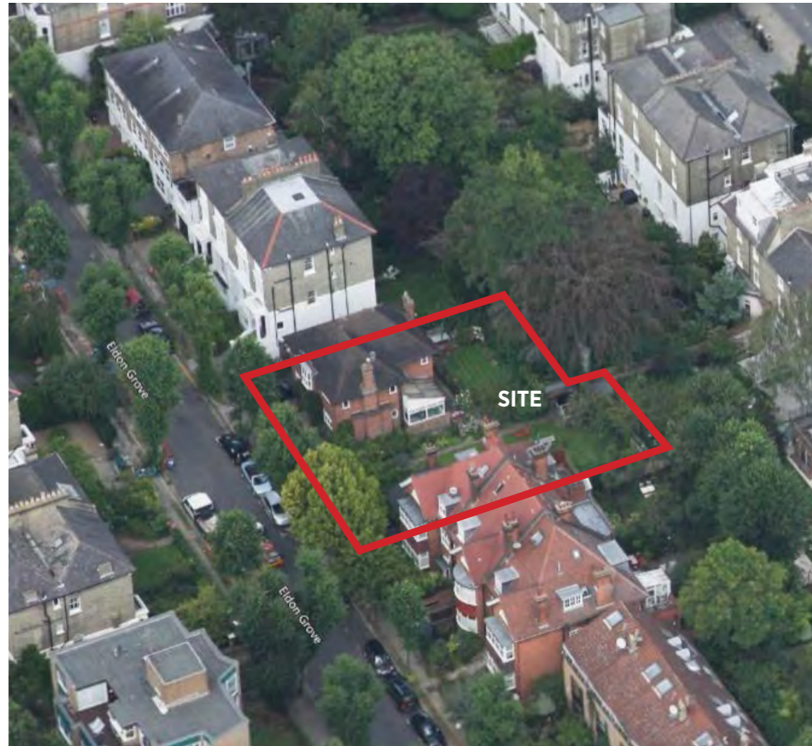
Front Aerial View
