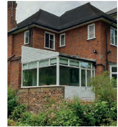
Existing photograph of the 'untidy' rear facade / conservatory
