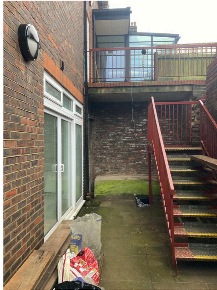
Photo 4: Looking South within lightwell
