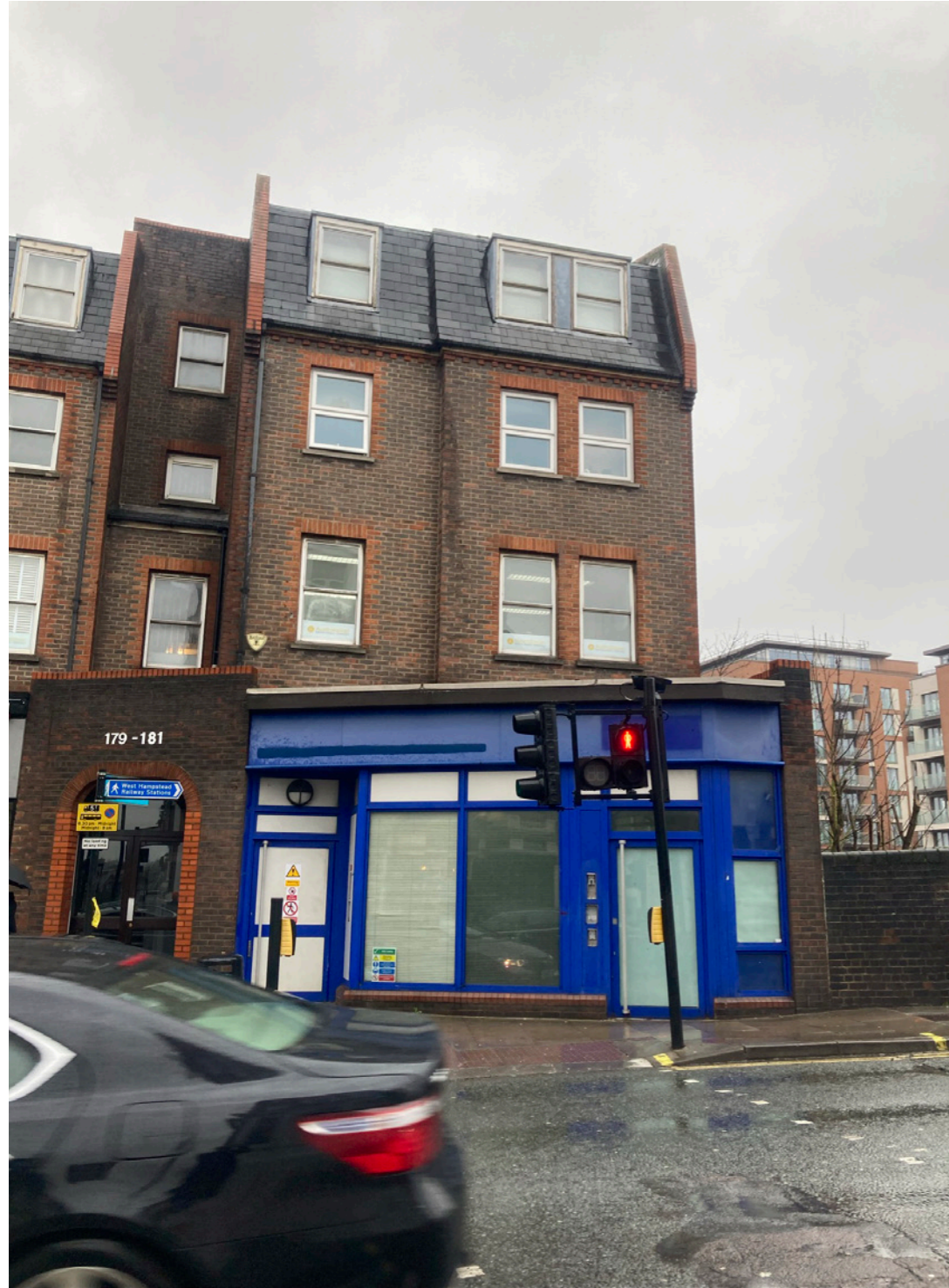
2 - Facing East and front facade of 179-181 West End Lane
