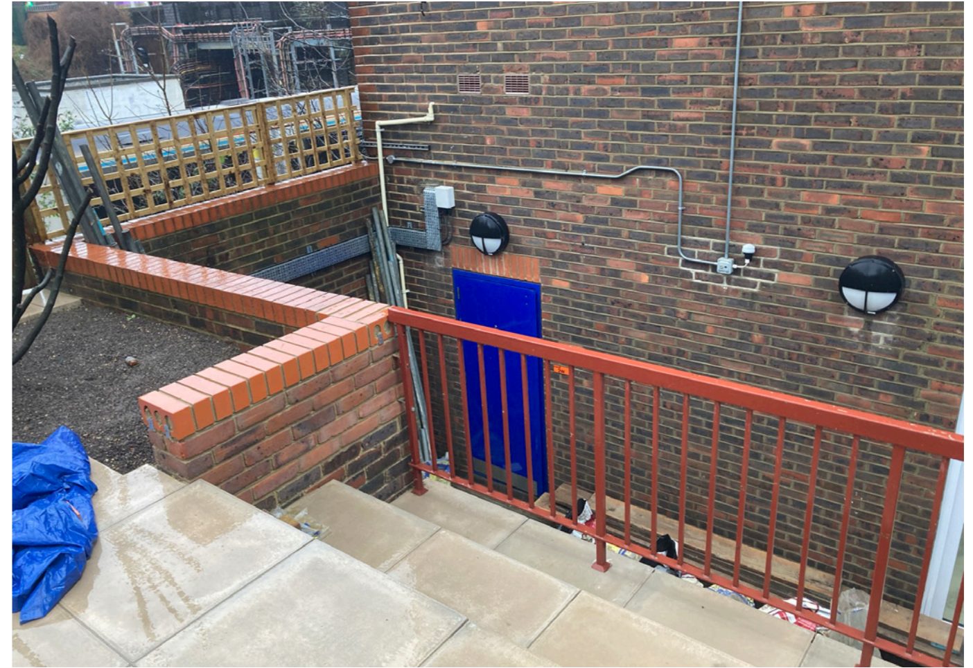
Photo 5: Looking West back towards lightwell from raised area beyond lightwell.
