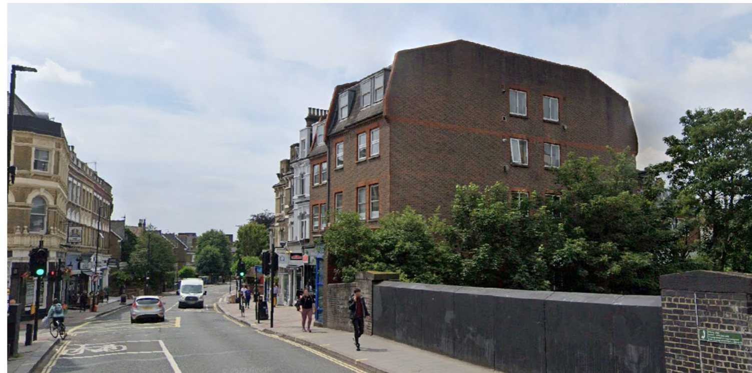
1 - Facing South along West End Lane. Flank of 79-181 shown on right hand side of image.
