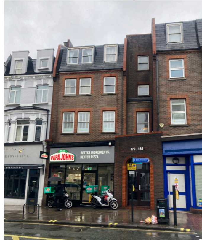
1 - Remaining front facade of 179-181 West End Lane
