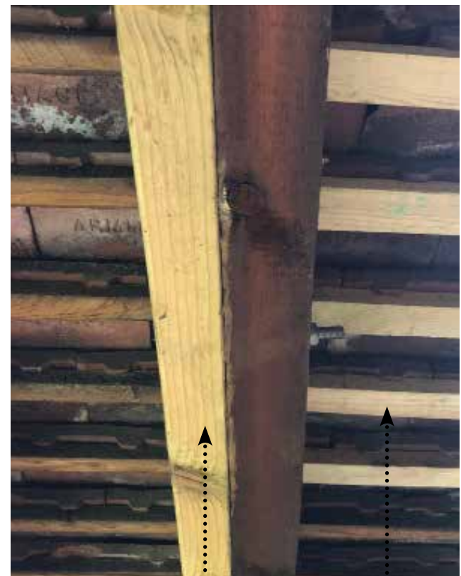
Absence of membrane, replacement timbers
