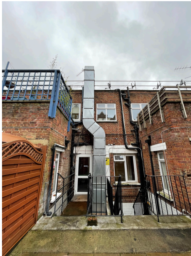
Picture 5 : Back view of building
