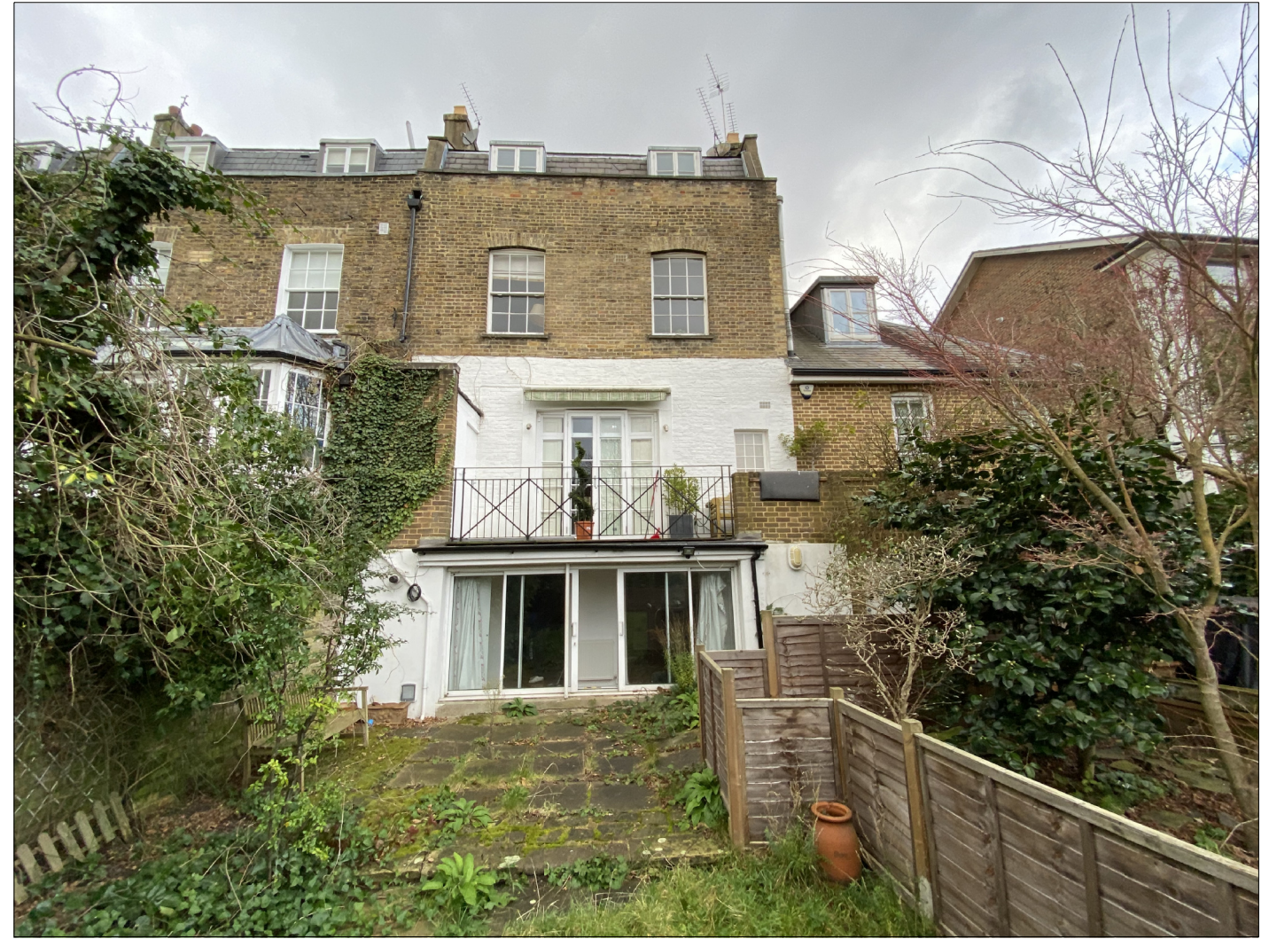
Existing View of Rear Elevation
