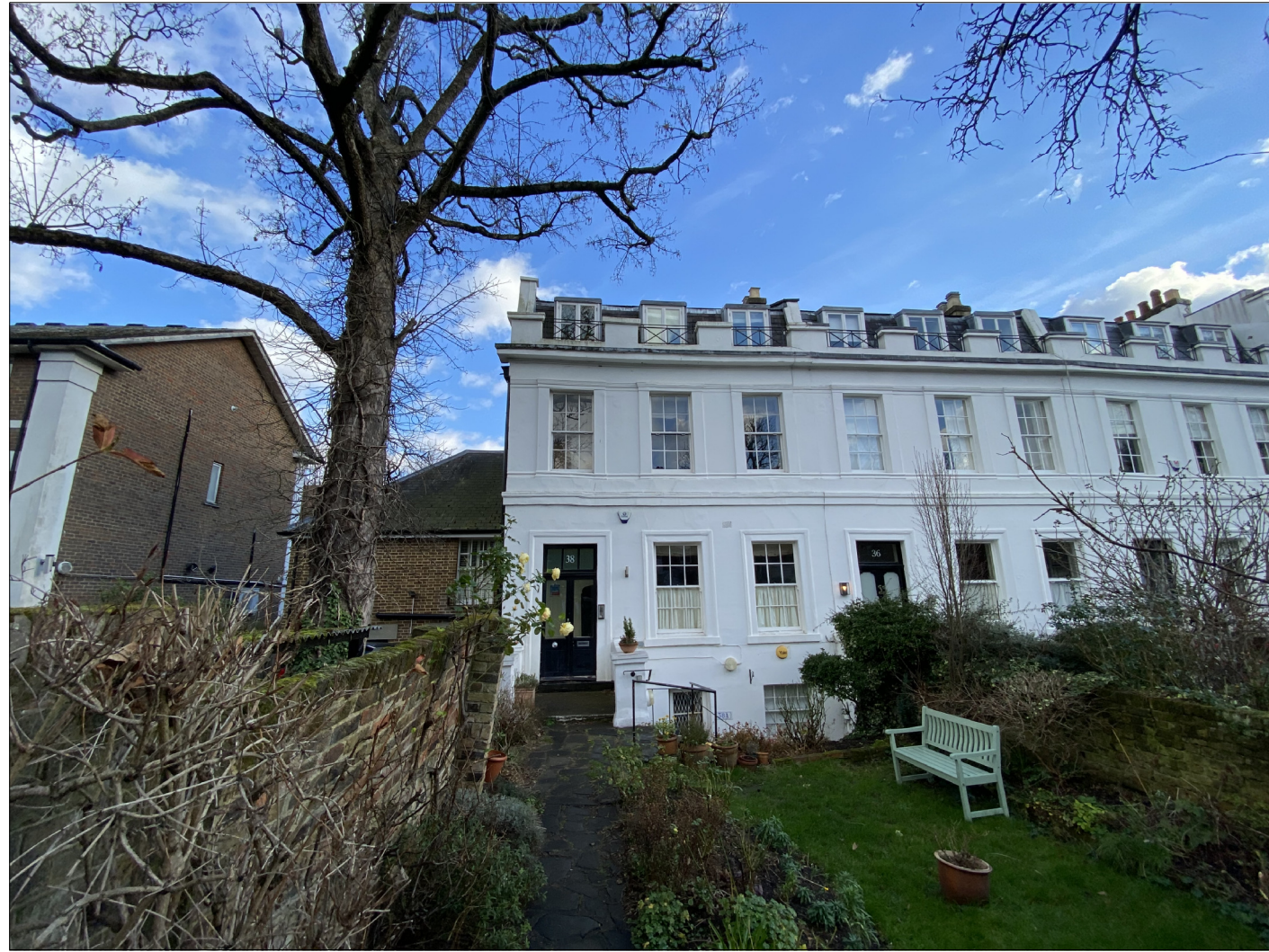
Existing View of Front Elevation
