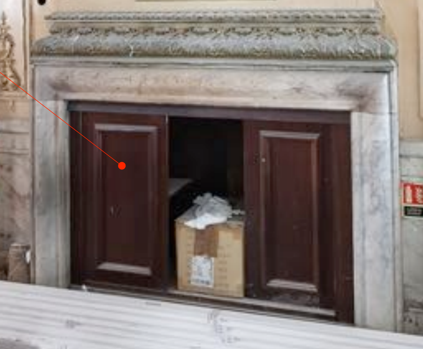
Joinery (timber doors) to be removed and fireplace re-instated
