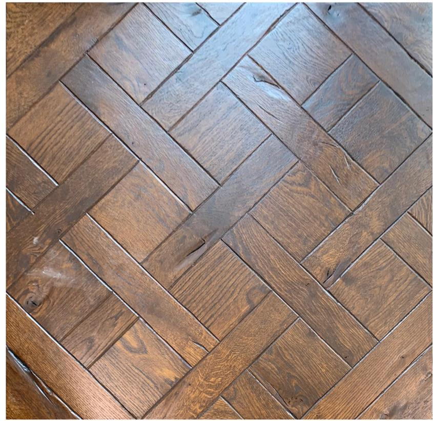
FPS Flooring LTD. Latimer Rd, London, W10 6QW Ref: HY/PDV-ANT-MAH-COSTA Continuous Versailles Design (i.e. no border panel) NBS spec: K20/110/Type A
